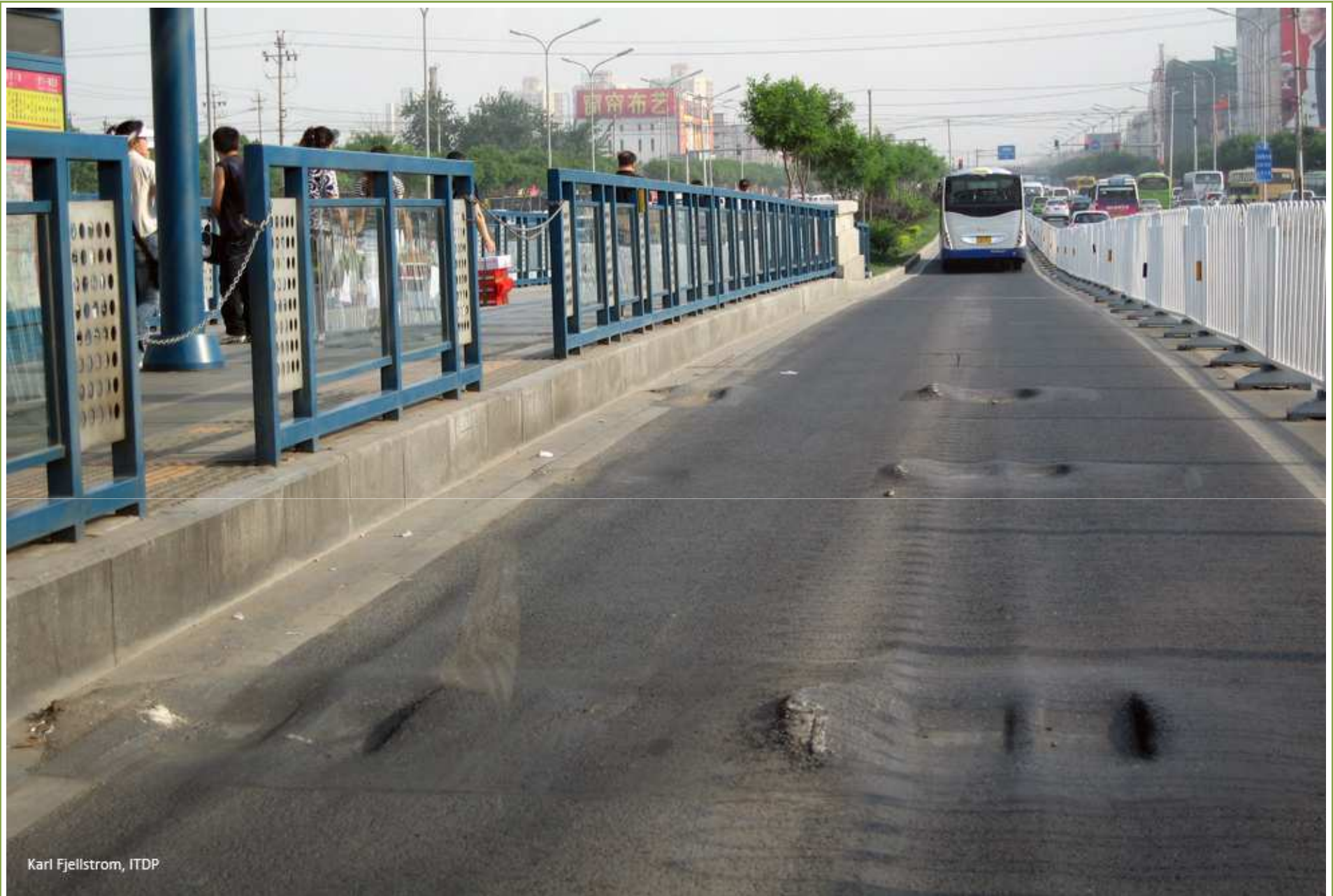
Runway degradation in corridor 1
