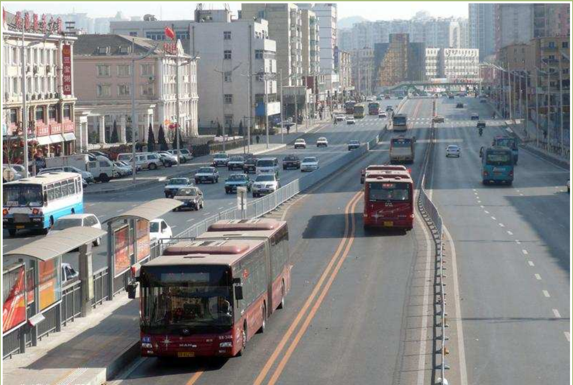
Median aligned busway; minimal cover at stations; low demand along the corridor
