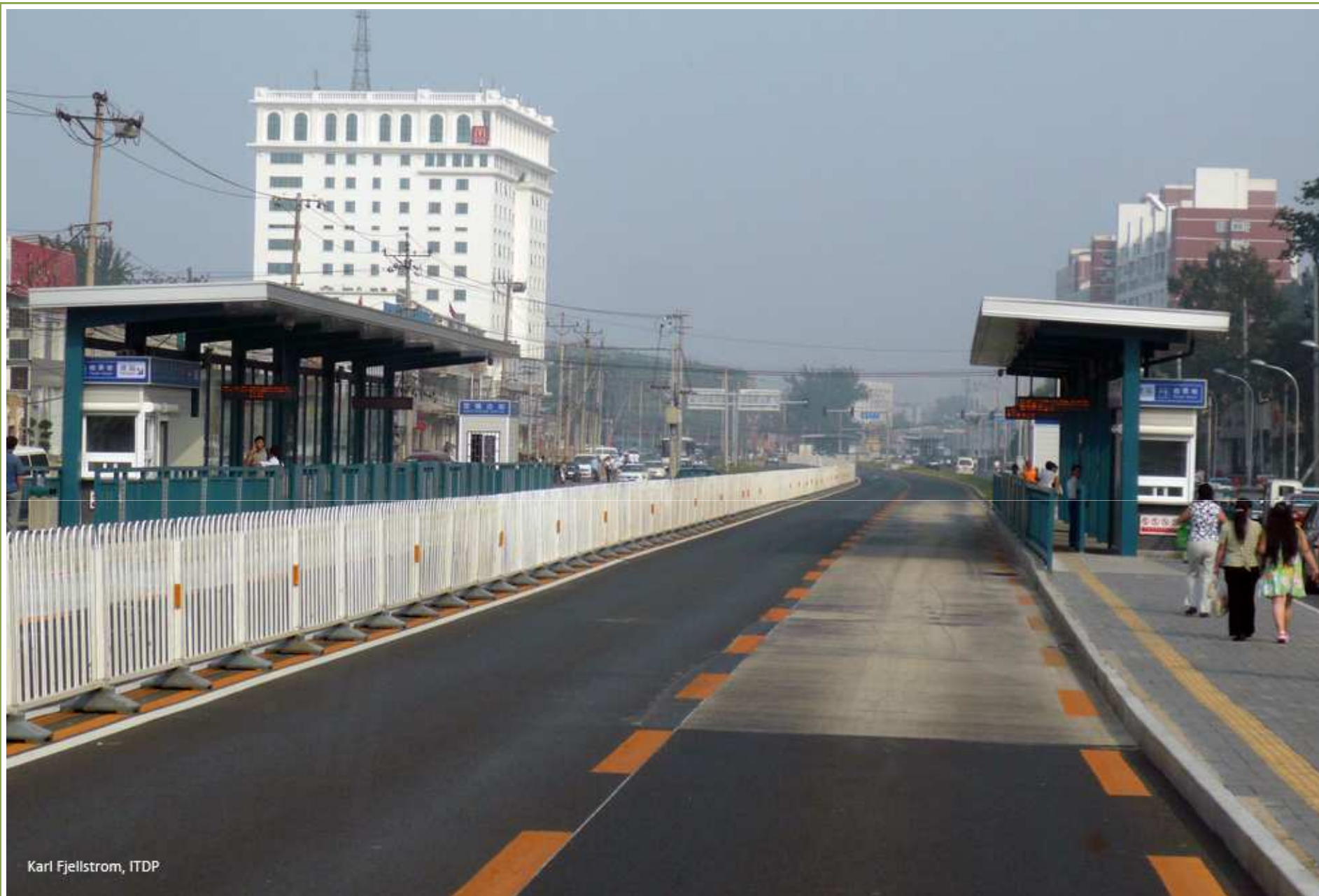
Better stations in outer part of corridor 2; overtaking mixed traffic; right-side doors
