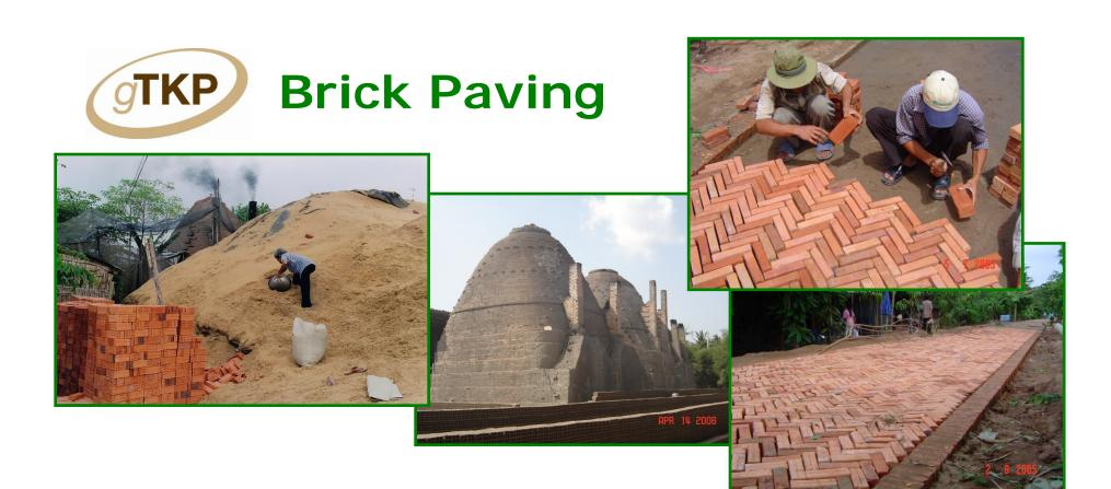
Burnt Clay Brick paving can be an important option in areas lacking hard stone resources, for example in delta regions. The clay can be fired to high quality bricks using small scale kilns and renewable energy sources, such as waste rice husk. Materials haulage can be minimized and local employment created in brick production for roads and building construction.
