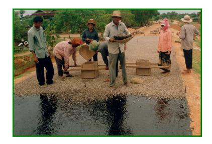
A range of surface and paving options is available using bitumen as a seal or binding material. They can be particularly suitable for labour based methods if emulsions are used. Techniques include 'chip' seals, sand seals, Ottaseals, and bitumen macadams. The thin seals will require suitable pavement layers to be constructed between the road foundation and surface.
