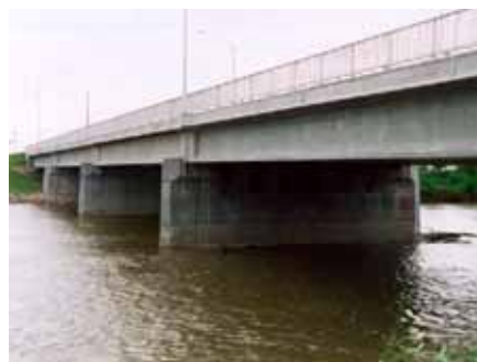
Figure 12.7: Pre-stressed beam and slab bridge
