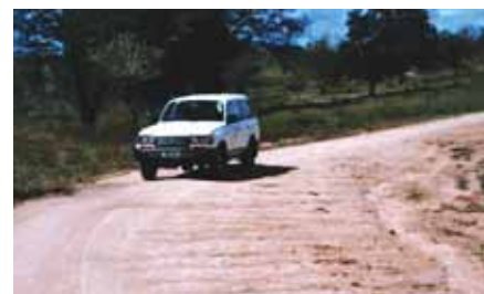
Figure 11.1: Transverse erosion on a super-elevated curve
