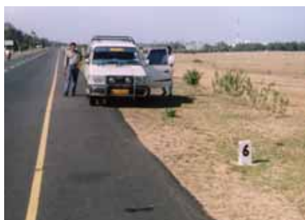
Figure 11.2: Sealed shoulders together with low embankment slopes ensure that the pavement remains dry and strong.
