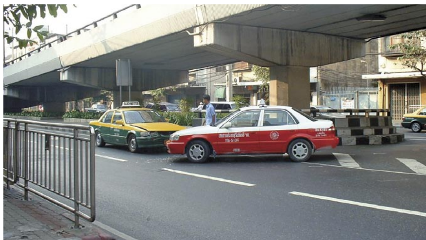
Fig. 5 A combination of low cost measures described in Table 1 – better channelisation, medians and traffic signs, for example – could have averted this accident in Bangkok, Thailand, which was caused by confusion surrounding a contra-flow bus lane.
