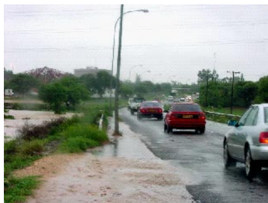
Fig. 6 A road in Gaborone, Botswana without surfaced sidewalks. Pedestrians are forced to walk on the road after rain.
