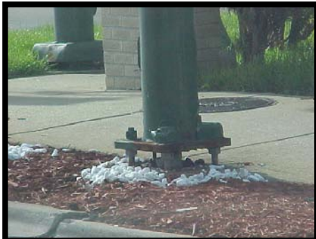
Slip base design breakaway post
