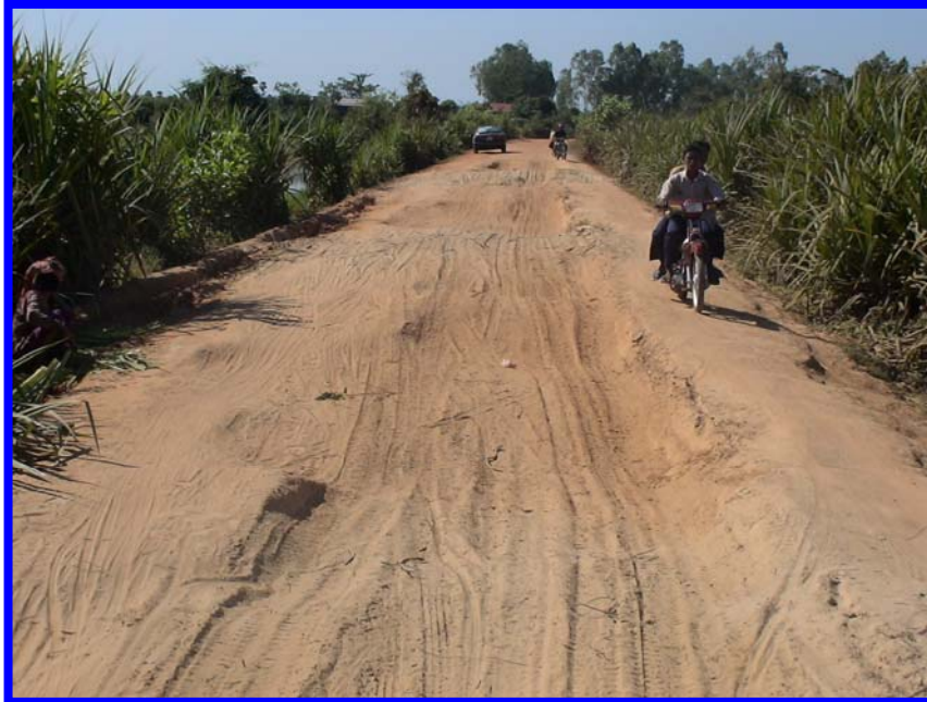
Figure 1 – A donor funded project gravel road within 2 years of maintenance cessation (photographed in the dry season! – impassable to motor cars)
