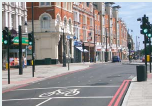
Fig. 2.14 Clapham High Street – new street layout. The carriageway has been narrowed from three to two lanes and guardrailing has been removed.
