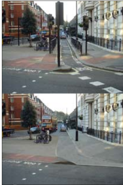
Fig. A3.5 Existing and modified photo showing the visual impact of removing pedestrian signals, road markings and guardrailing.
