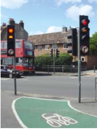
Fig. 3.10 Cycle crossing at signalised junction – only one primary signal head is required.
