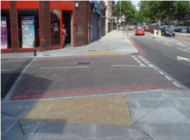
Fig. 3.3 A simple raised junction entry which uses a standard palette of relatively low-cost materials.
