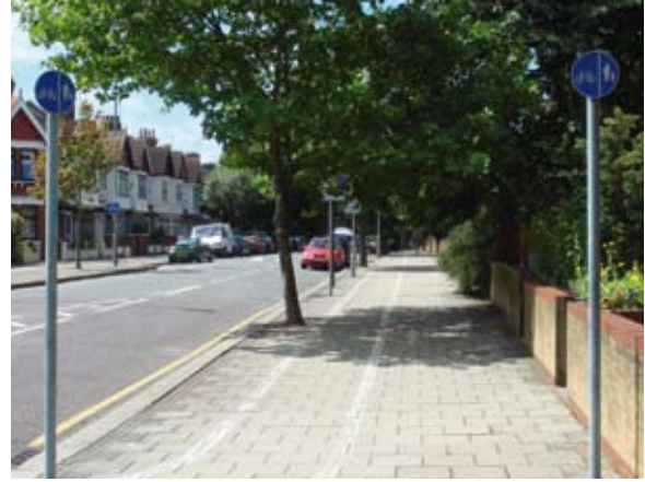
Fig. 3.12 Segregated cycle path – two signs excessive for this lightly-trafficked route.
