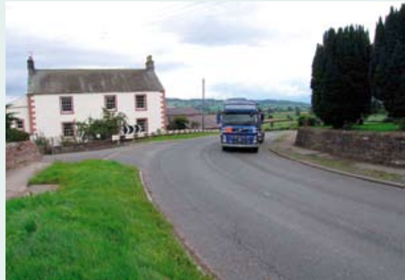
Fig. 2.12 A6 Clifton Village – after. Carriageway narrowed and road centrelines removed.
