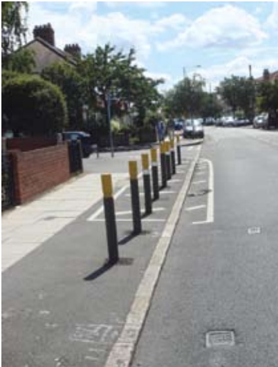
Fig. 3.7 Ad-hoc measures to prevent parking on the footway – could the bollards and lines be reduced, or replaced with double yellow lines?
