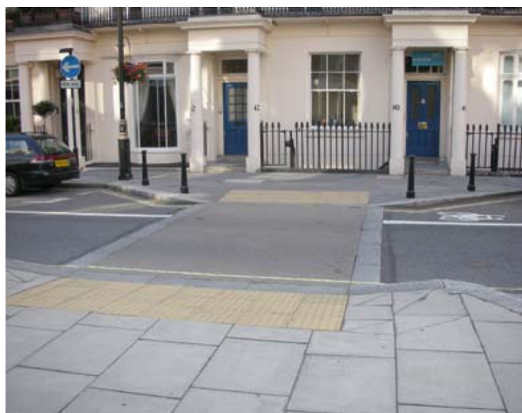
Fig. 3.19 This raised junction entry and informal crossing have been designed sensitively in recognition of the historic character of their surroundings.
