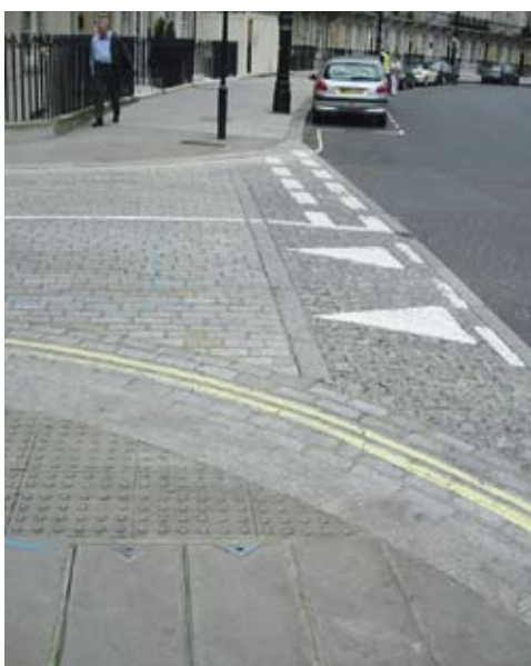
Fig. 3.19 This raised junction entry and informal crossing have been designed sensitively in recognition of the historic character of their surroundings.
