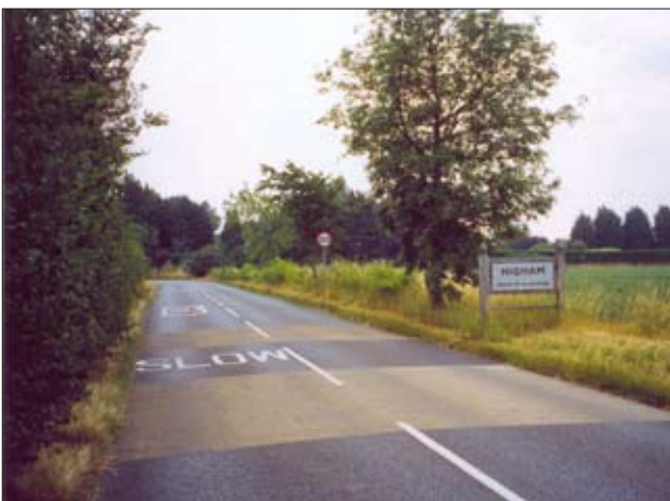
Fig. 3.13 Village gateway treatment – subtle measures used in accordance with Suffolk’s stated policy in The Suffolk Countryside Manual, 2003 . The hedgerow on the left was planted with the purpose of giving the impression of a narrowed carriageway.
