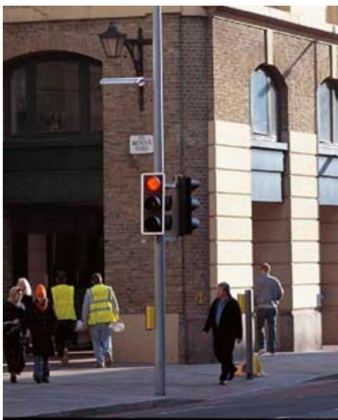
Fig. 3.1 Pelican crossing – signal heads mounted onto existing lamp column to reduce clutter, though a second push button mounting pole is provided, adding to street clutter.
