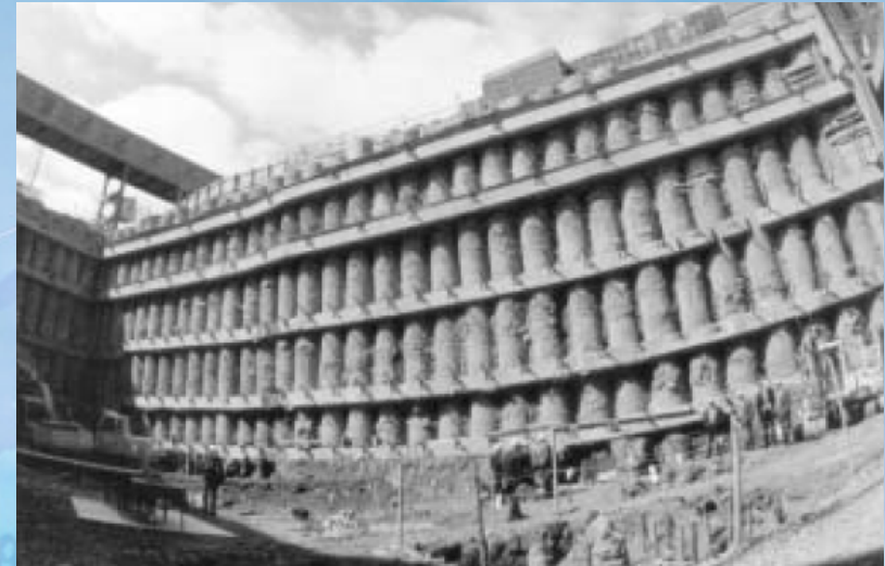
Anchored contiguous piled wall
