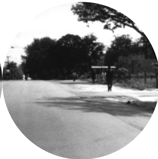
Old Dar-es-Salaam road, Morogoro, immediately after reconstruction in 1999
