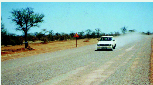
Aggregate dislodged by traffic should be broomed back into the wheel paths. This is to ensure maximum embedment of the aggregate into the soft binder.
