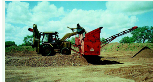
The wide grading envelope allowed for the Otta Seal maximises the use of natural gravel (as-dug material), which in many cases requires only screening of oversize materials by use of a power screen (Mahalapye – Machaneng road).
