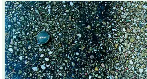
After some 8 - 12 weeks, depending on traffic, the aggregate becomes embedded and a “premix” like appearance starts to appear.
