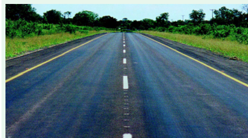
After some months of trafficking, the Otta Seal “beds down” and provides an uniform appearance similar to asphaltic concrete (Kasane – Ngoma road).
