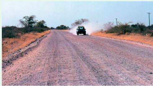
Unsealed roads very often corrugate, resulting in a rough surface and associated high maintenance and operational costs.
