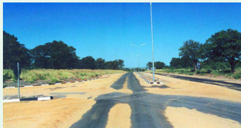
The sand blown off by traffic should be broomed back into the exposed areas until full embedment is achieved.
