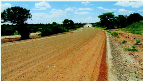
An Otta Seal surfacing 2-3 days after construction.
