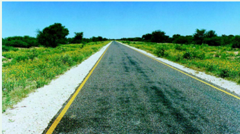
A single Otta Seal with a sand cover seal on the Kang – Hukuntsi road. After more than 9 years in service and without any surfacing maintenance the surfacing performs excellently.
