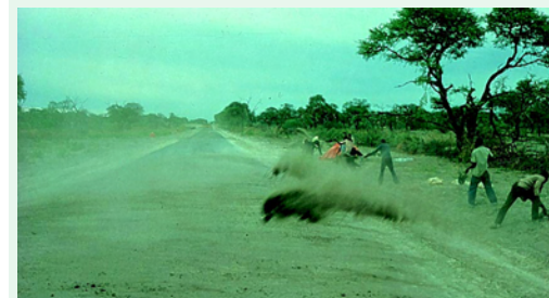
The aggregate requirements for sand cover seal are very relaxed. Kalahari sand directly from the road reserve area can be used successfully for this purpose (Sehitwa - Tsau road).
