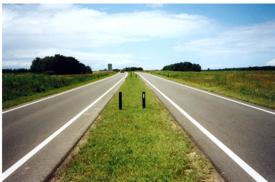
Distributor road, dual carriageway, one lane
