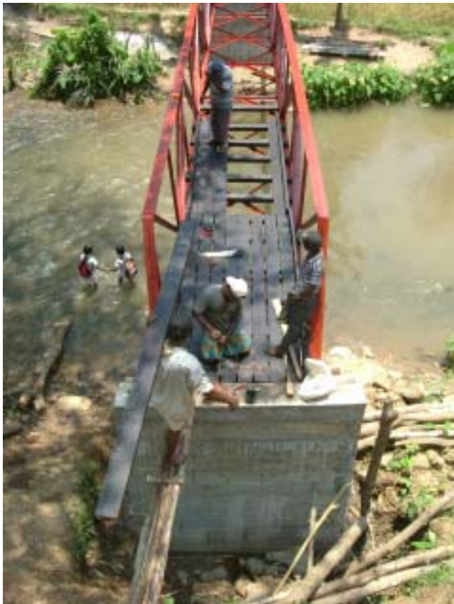
Figure 4.16: Assembly of Deck
