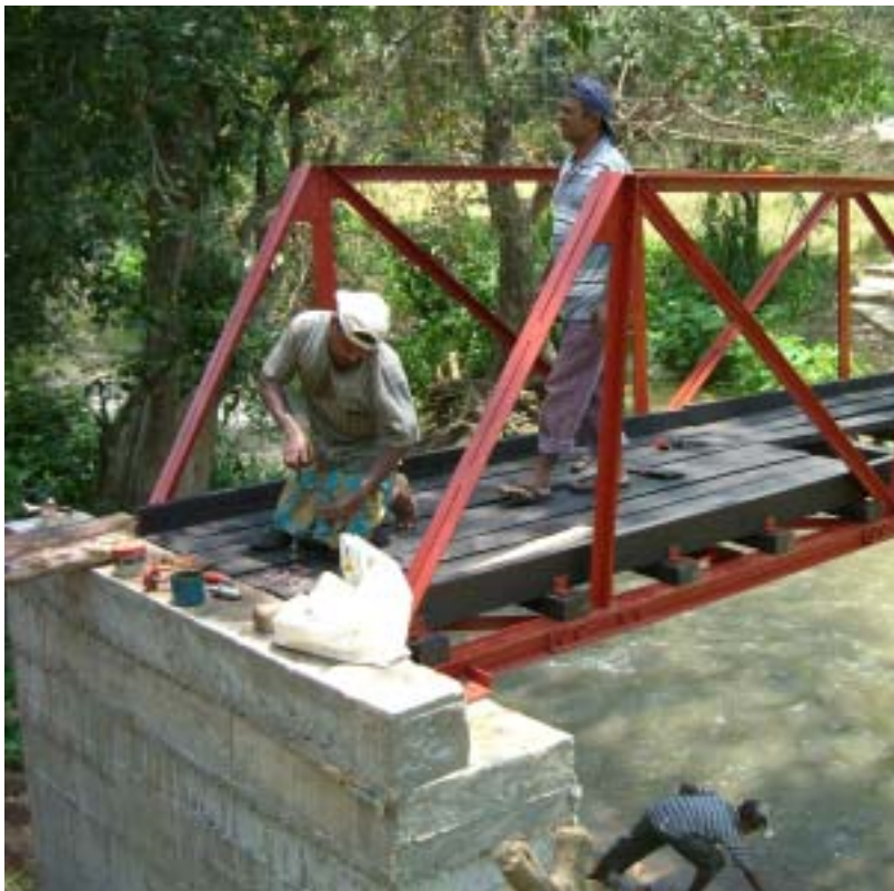
Figure 4.15: Fitting the Decking
