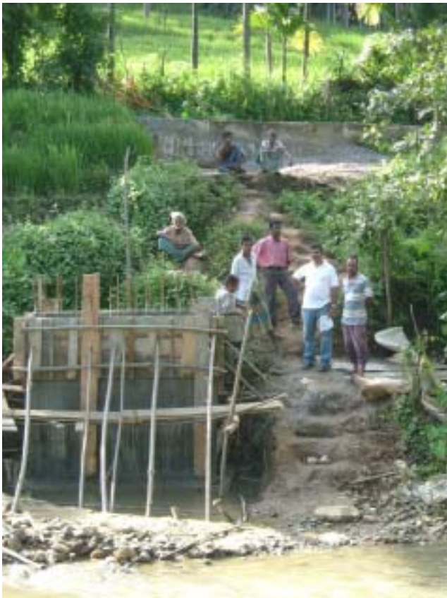
Figure 4.2: Construction of the Abutments
