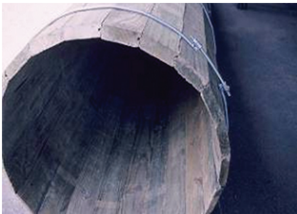
Figure 9.13 Timber stave culvert
