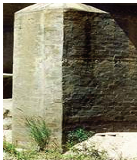
Figure 8.61 Brick pier
