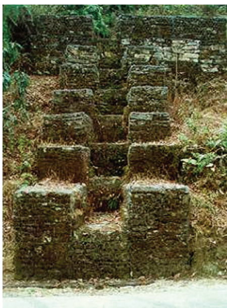
Figure 8.45 Gabion basket step waterfall
