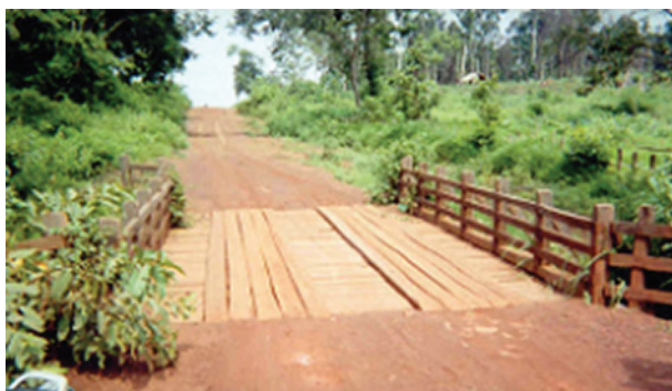
Figure 8.63 Timber bridge with handrails
