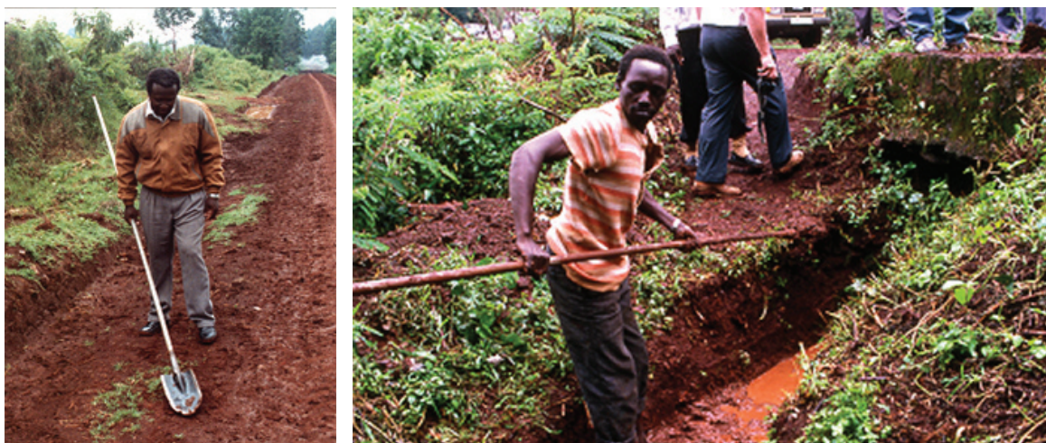
Figure 10.1 and 10.2 Culvert cleaning tool
