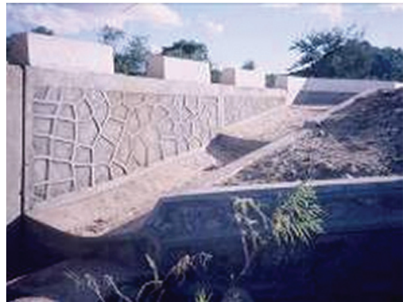
Figure 8.38 Masonry side drains at the edge of an approach way to prevent erosion
