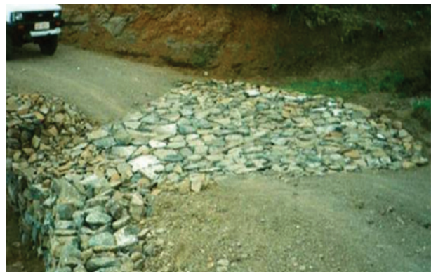
Figure 8.7 Hand pitched stone drift
