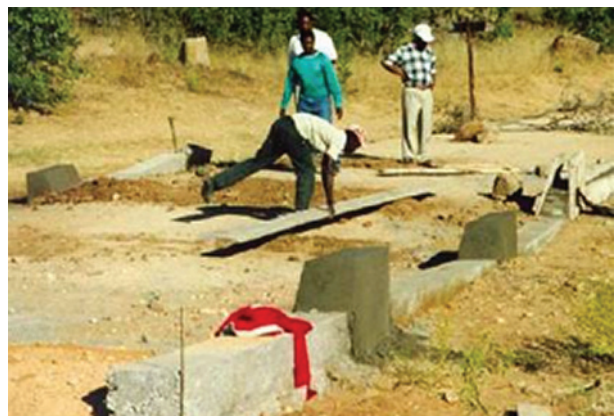
Figure 8.5 Guide stones at the edge of a drift
