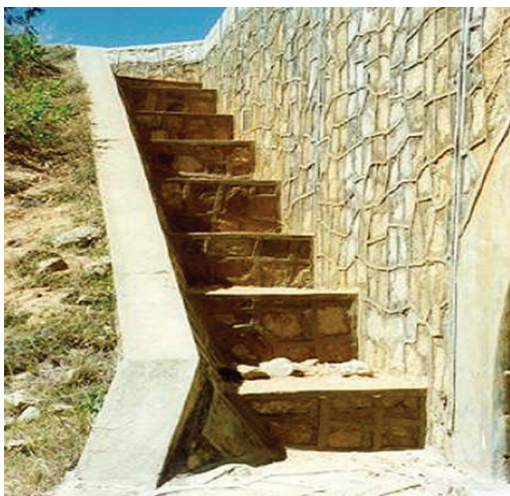
Figure 8.32 Wingwall cascade
