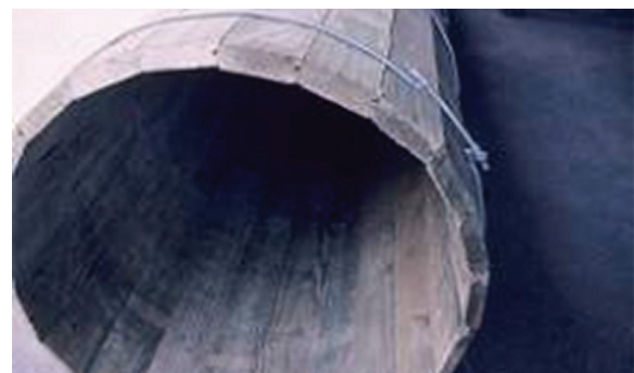
Figure 8.17 Timber barrel culvert
