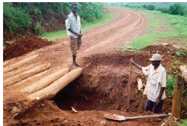
Figure 8.19 Timber pole culvert during reconstruction
