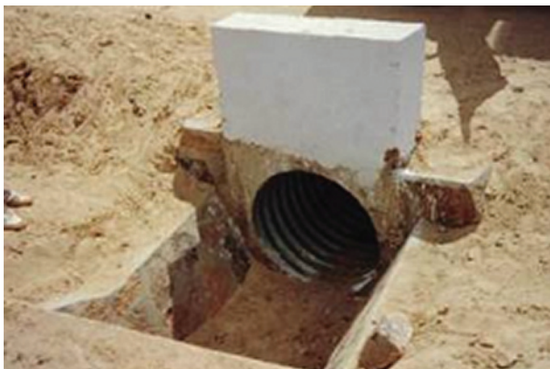
Figure 8.26 Drop inlet on stream culvert
