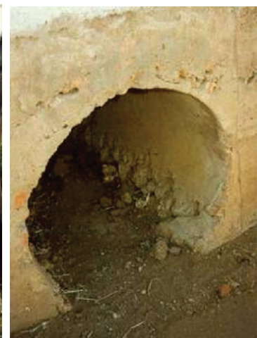
Figure 8.21 Cast in situ culvert
