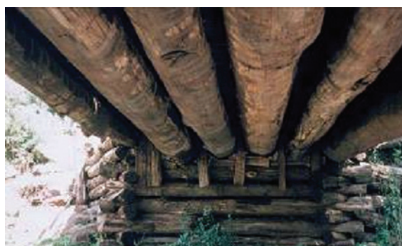
Figure 7.43 Log abutments & deck
