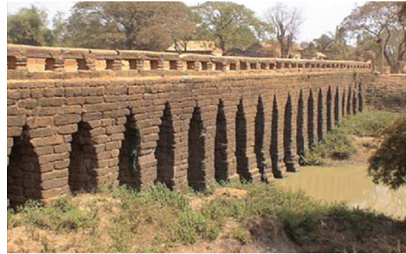
Figure 7.2 Dry jointed, laterite, stone viaduct, approximately 1,000 years old, still in service on a national main road.
