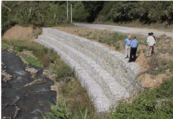
Figure 7.22 Gabion retaining wall used as river bank protection
