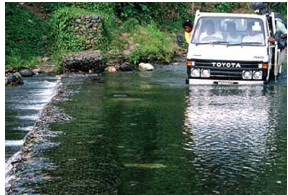
Figure 7.25 Gabion river crossing
