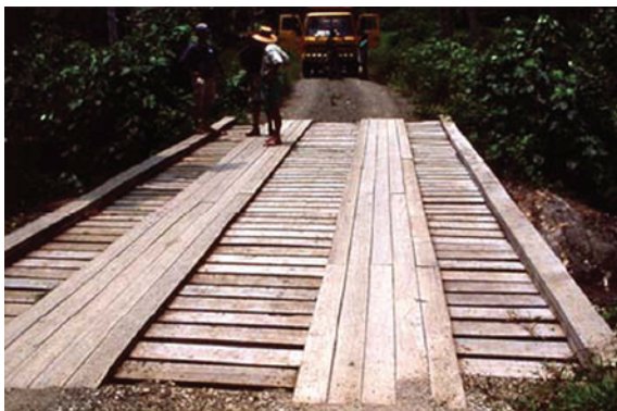
Figure 7.35 - Completed timber deck
