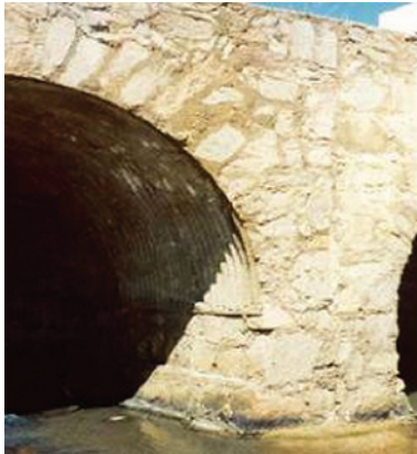
Figure 7.8 Rubble stone large bore culvert
