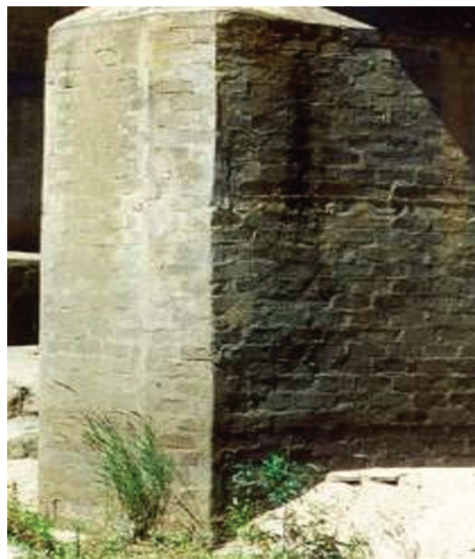
Figure 7.32 Bricks in a bridge pier
