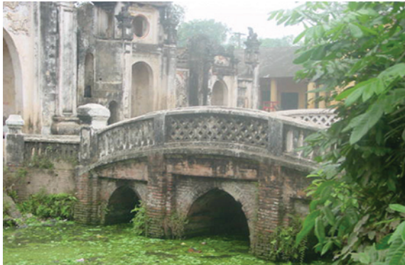
Figure 7.27 - Fired clay brick structures exist in many countries and still provide service for today's traffic after centuries of use.
