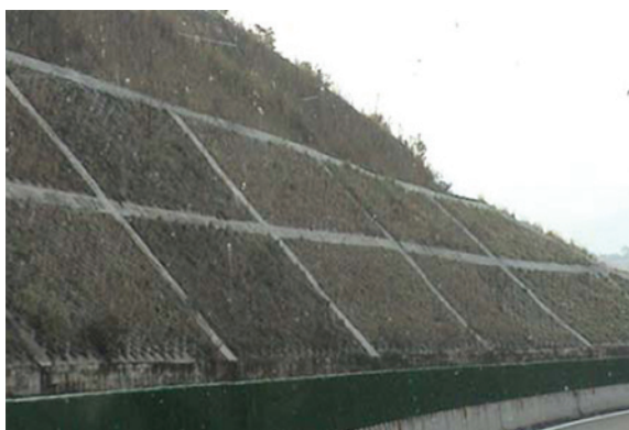
Figure 7.15 Hybrid retaining wall
