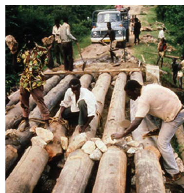
Figure 7.39 Timber poles as deck beams of a twin span bridge
