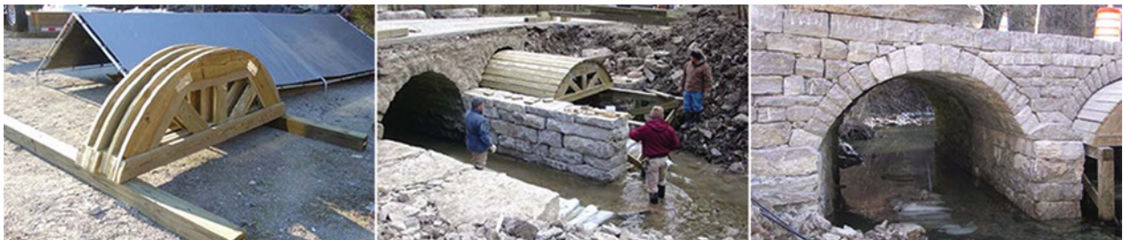
Figures 7.18 Dry stone masonry culvert extension works – Dry stone Conservancy, USA
