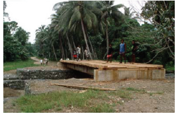
Figure 7.34 - Timber deck on recycled steel beams
