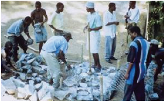
Figure 7.21 Filling gabion baskets
