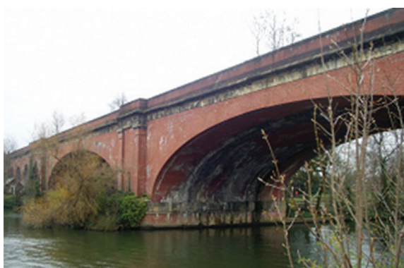
Figure 7.26 - Fired clay brick is a very versatile material. This elliptical brick arch bridge over the River Thames at Maidenhead, UK was constructed in 1838 and has two main spans of 38 metres. It is still in use today (designer: Isambard Kingdom Brunel) photograph by Jon Combe
