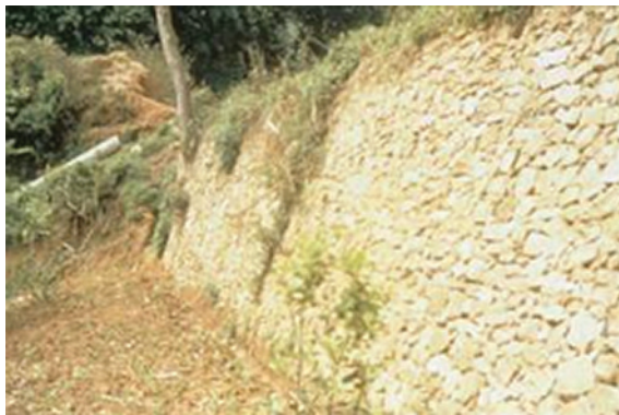
Figure 7.13 Dry stone wall supporting road embankment
