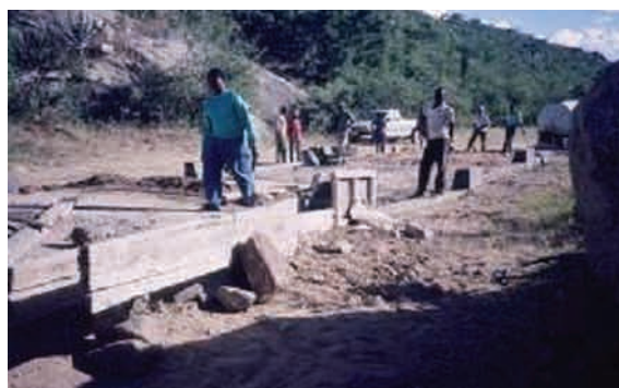
Figure 7.52 Concrete drift in construction
