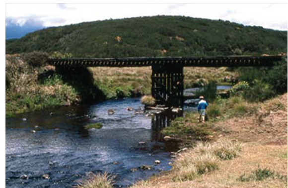
Figure 7.36 - Timber bridge deck, pier and abutments
