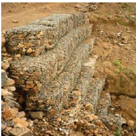
Figure 7.19 Gabions supporting a road on a steep slope
