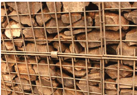
Figure 7.24 Steel mesh gabions
