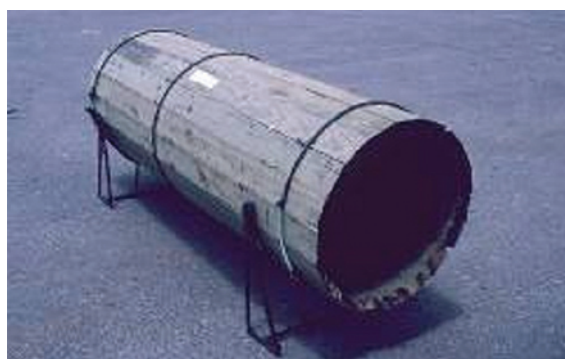
Figure 7.44 Treated timber culvert
