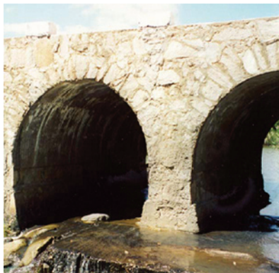
Figure 4.11 Large bore arch culverts
