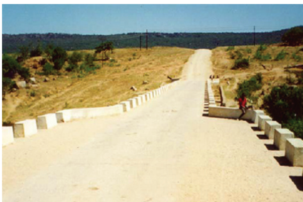
Figure 3.4 Guide stones narrowing road width
