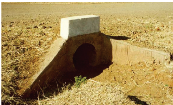
Figure 3.5 Culvert head stone outside main running lanes
