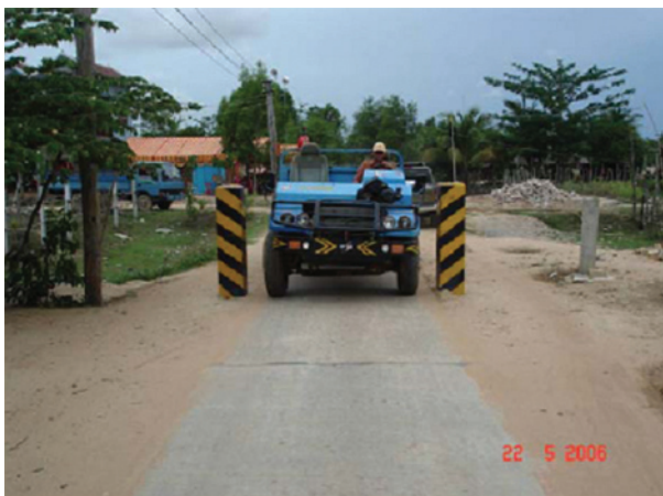
Figure 3.2 Robust width restrictions can be used in some instances to restrict heavy vehicles
