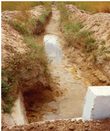
Figure 5.8 Long culvert outfall
