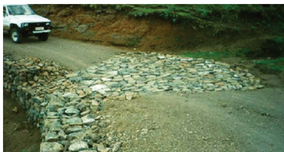
Figure 4.3 A basic hand packed stone drift
