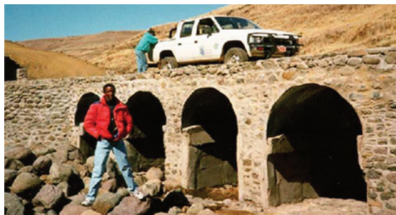
Figure 4.15 Is this a vented ford or a multi-bore culvert?
