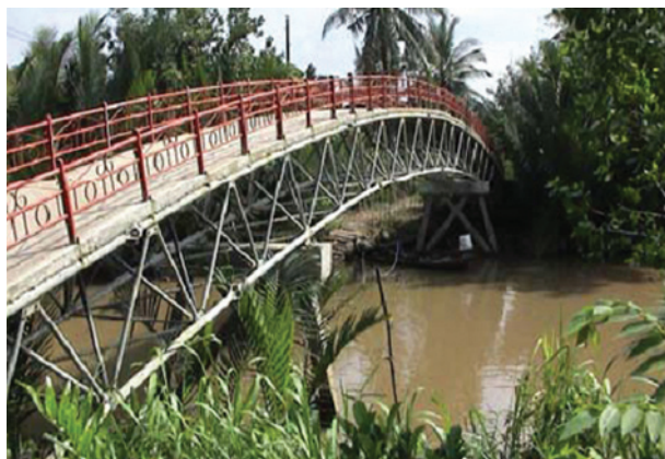
Figure 1.1 Steel lattice bridge for motorcycle traffic
