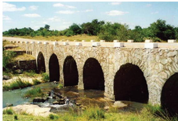
Figure 4.12 Guide stones on large bore culvert structure
