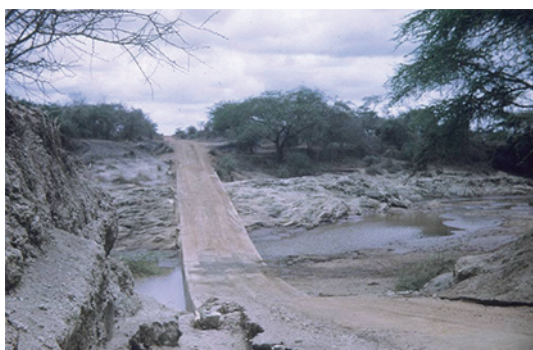
Figure 4.9 Concrete vented causeway
