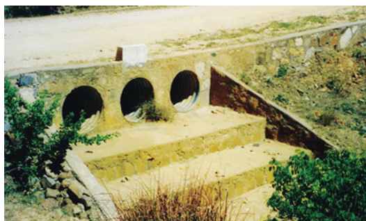
Figure 4.5 A three barrel corrugated steel culvert with stepped outfall apron
