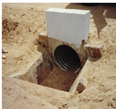
Figure 5.10 Culvert drop inlets
