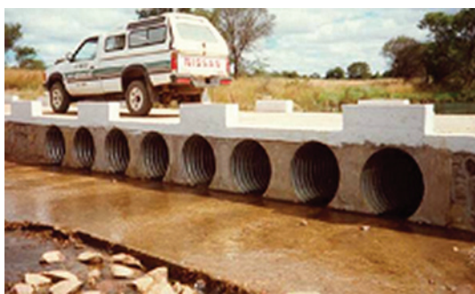
Figure 4.8 Downstream protection to a vented ford
