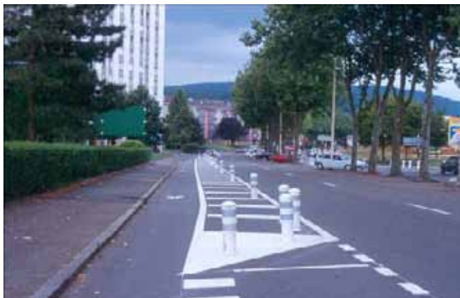
Figure 4.10. Temporary design in Belfort (France)
