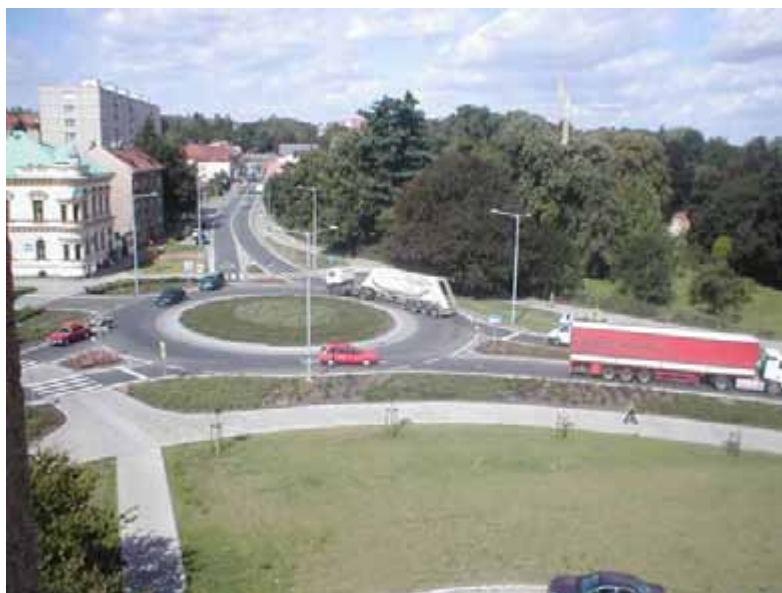
Figure 4.6. Roundabout in Chrudim (Czech Republic)
