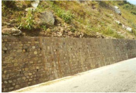
Mortared masonry wall
