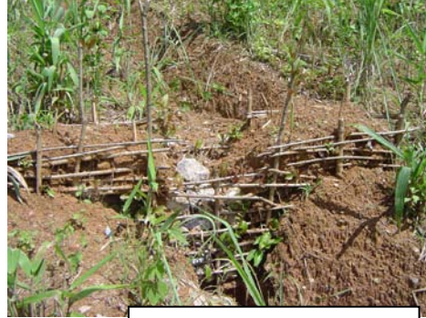
A small live check dam a few weeks after construction.
