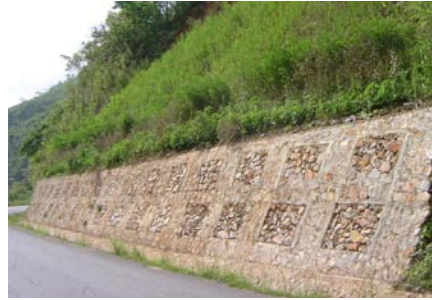
Composite masonry wall
