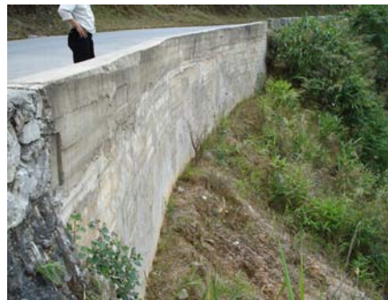
Reinforced concrete wall
