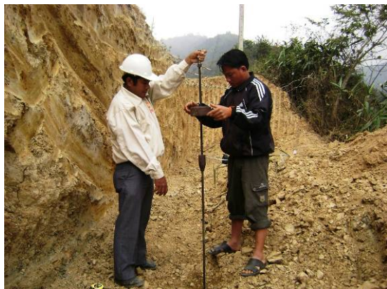
Figure 3-6: Dynamic Cone Penetrometer test
