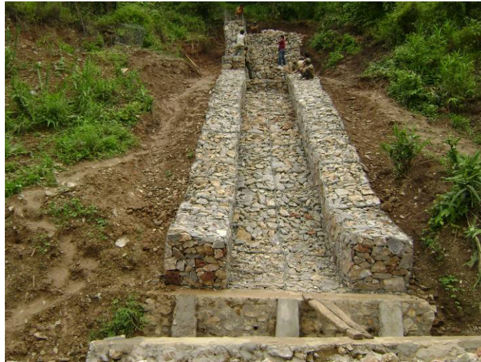
Figure 4-16. Typical gabion chute
