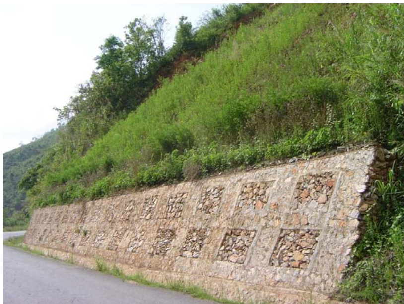
Figure 4-18: Typical bio-engineering measures to prevent surface erosion
