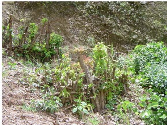
Figure 6-14: Live check dams about 3 months after completion, on a mixed debris slope
