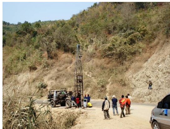
Figure 3-7: Site investigation using drill rigs
