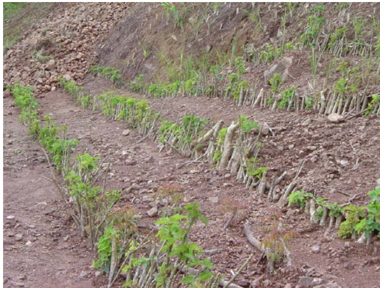
Figure 6-11: A palisade about 2 months after planting
