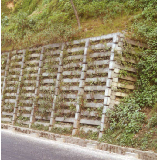
Concrete Crib Wall
