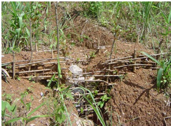
Figure 6-13: A live check dam on a soil slope, about 2 months after completion
