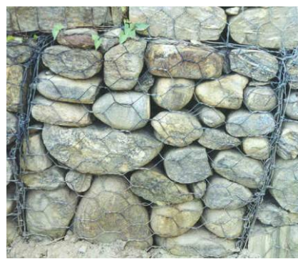
Figure 6-5: Examples of good and poor stone filling
