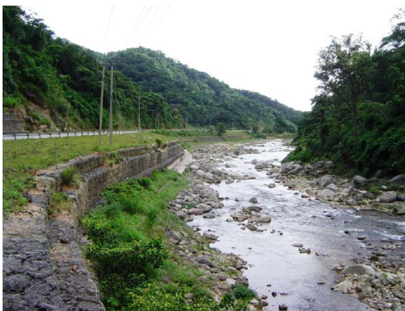
Figure 4-17. Typical gabion river training works
