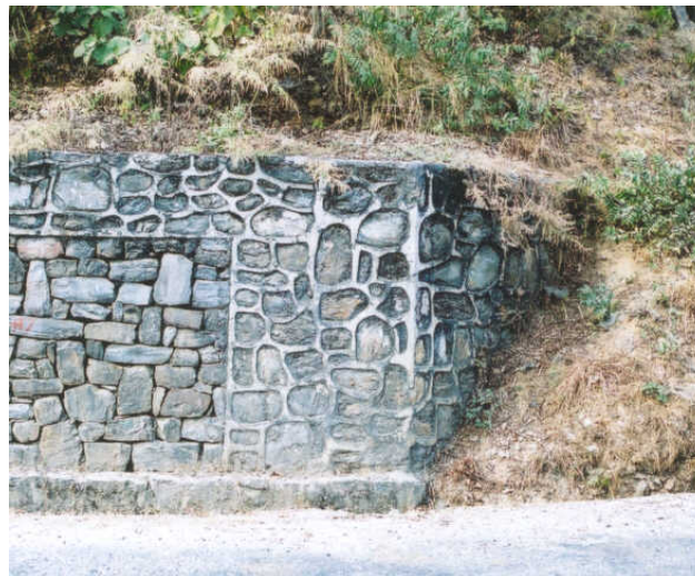
Figure 6.3: Retaining wall with angled return
