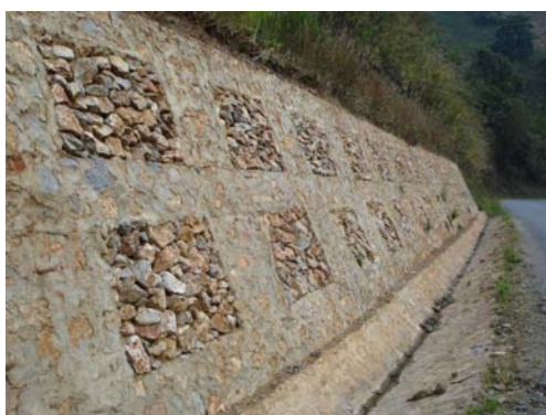
Figure 5-5: Typical composite masonry wall
