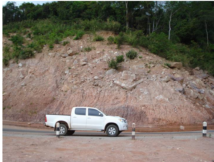
Figure 2-3: Shallow translational failure in colluvium
