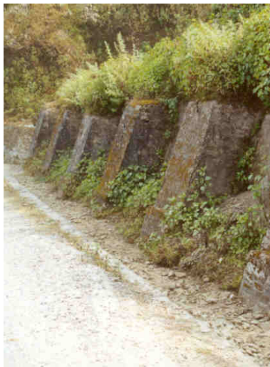
Buttressed mortared masonry wall
