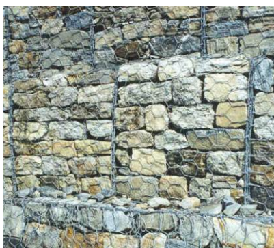
Figure 6-5: Examples of good and poor stone filling
