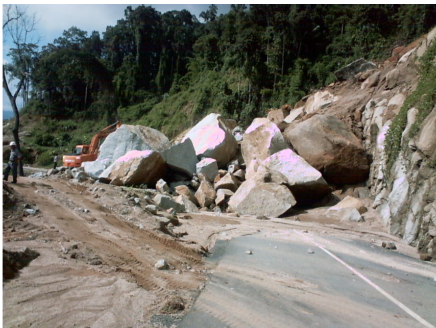
Figure 2-8: Rockfall on Road 18b
