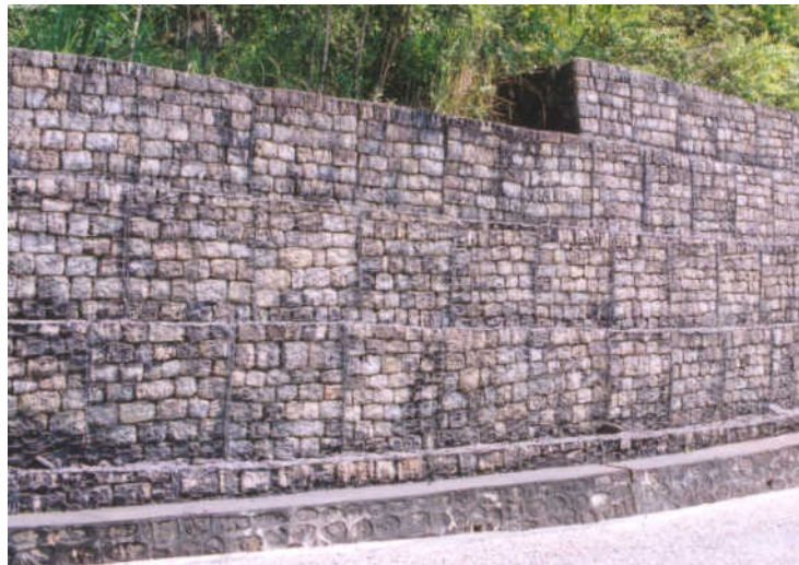
Figure 5-10: Typical gabion wall
