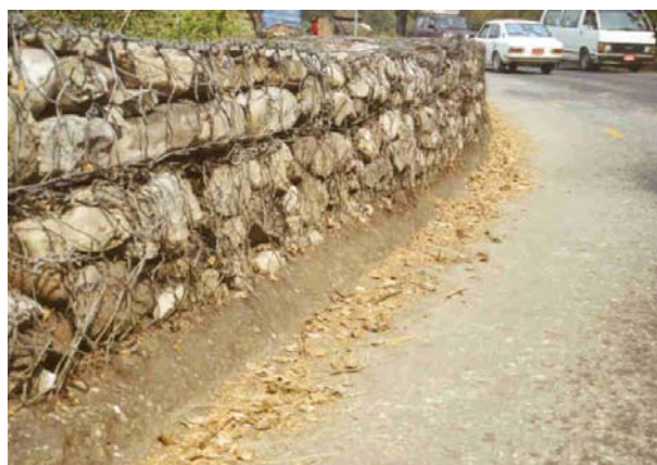
Figure 5-11: Bituminous upstand to gabion road supporting wall
