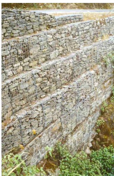
Figure 5-14: Gabion wall on stepped masonry base
