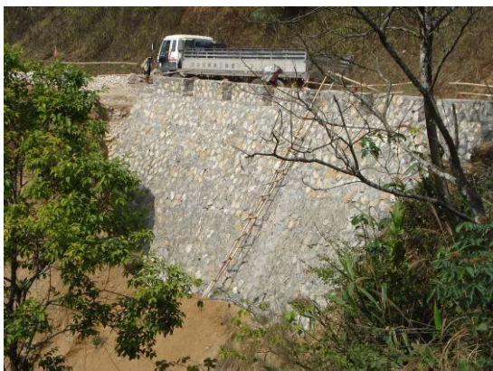
Figure 5-7: Typical mortared masonry wall
