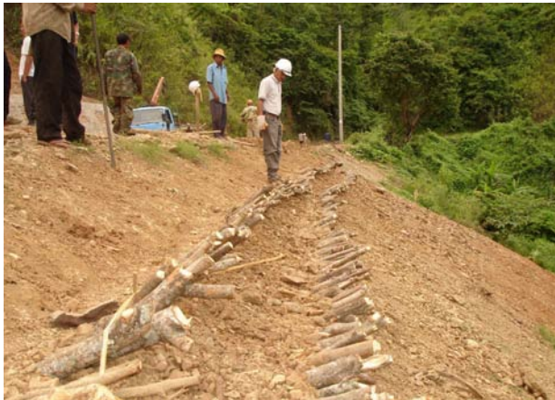
Figure 6-9: A freshly completed section of single-row brush layer
