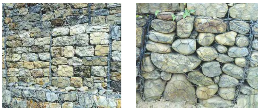
Figure 6-5: Examples of good and poor stone filling
