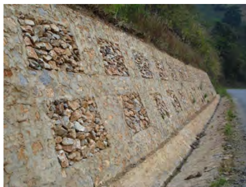
Figure 5-5: Typical composite masonry wall
