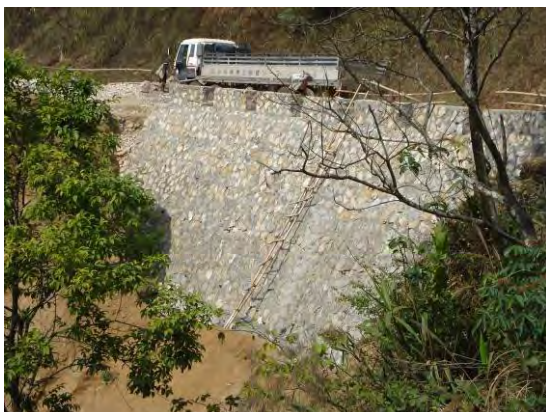
Figure 5-7: Typical mortared masonry wall
