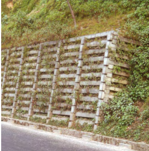
Concrete Crib Wall
