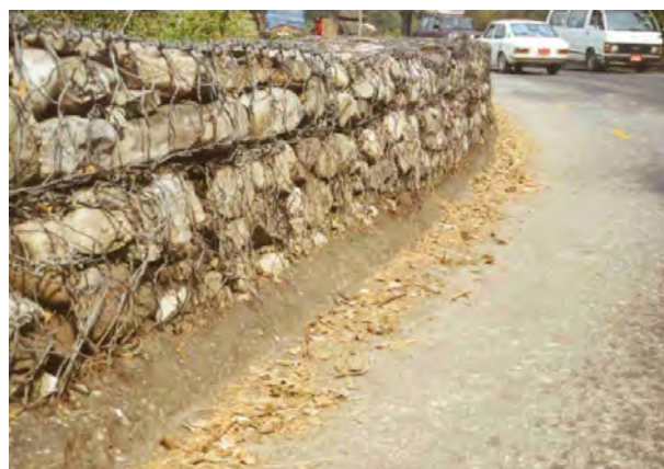
Figure 5-11: Bituminous upstand to gabion road supporting wall
