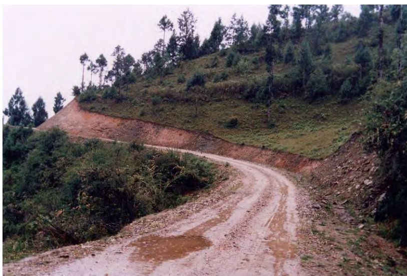
Figure B-2: Example of good cut slope construction
