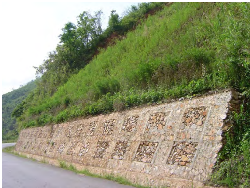
Figure 4-18: Typical bio-engineering measures to prevent surface erosion
