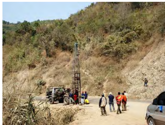
Figure 3-7: Site investigation using drill rigs
