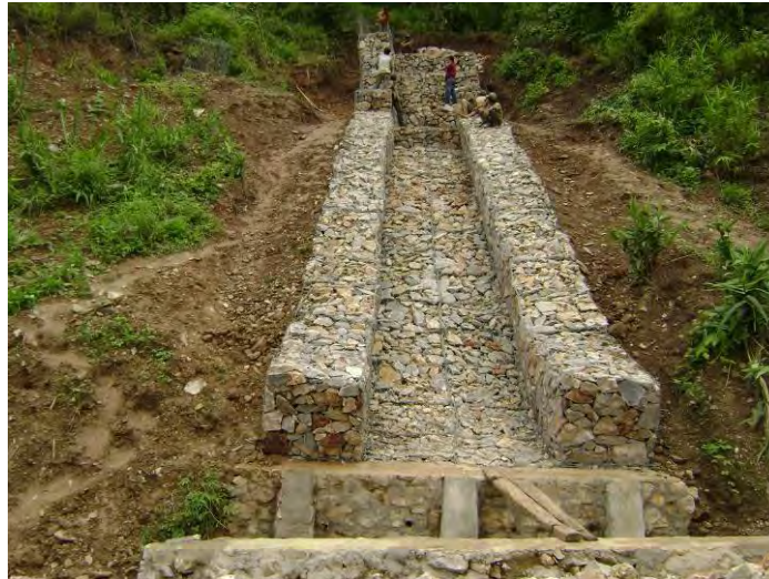
Figure 4-16. Typical gabion chute
