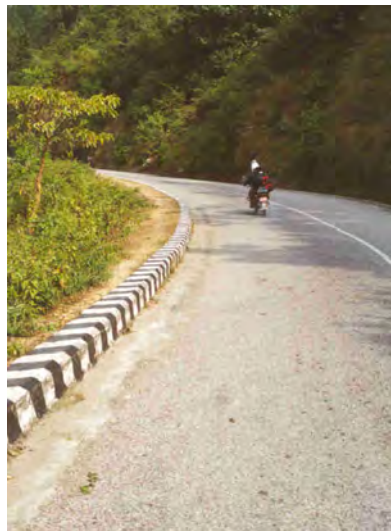
Figure 4-12: Kerb to road edge
