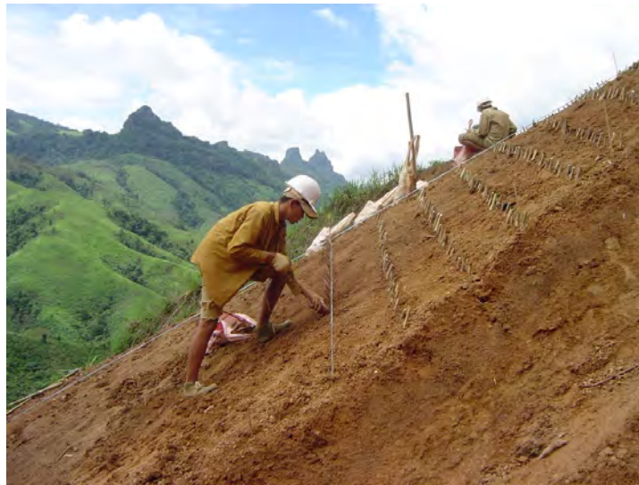
Figure 6-8: Planting lines of grass on a trimmed landslide head scarp
