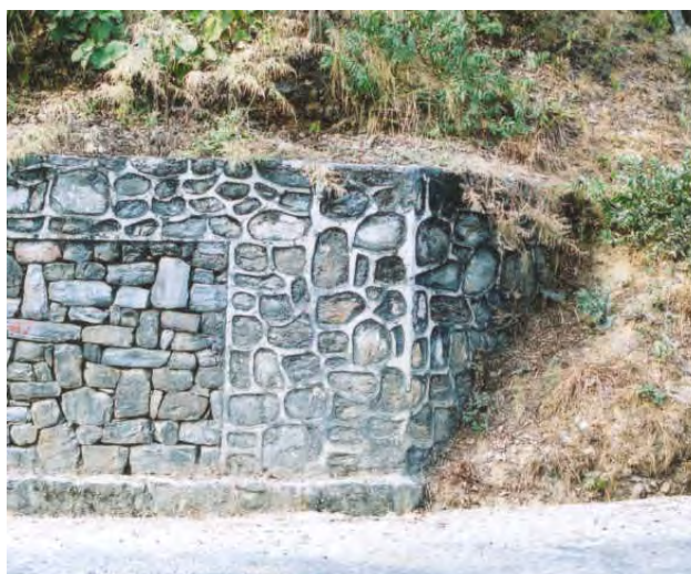
Figure 6.3: Retaining wall with angled return
