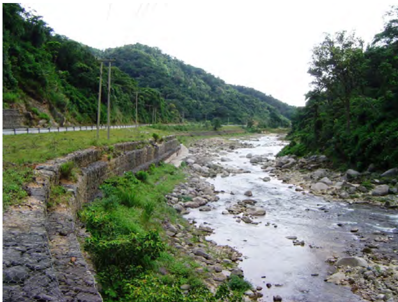
Figure 4-17. Typical gabion river training works
