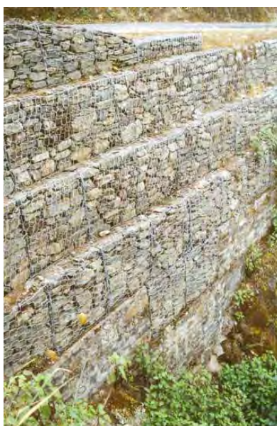
Figure 5-14: Gabion wall on stepped masonry base
