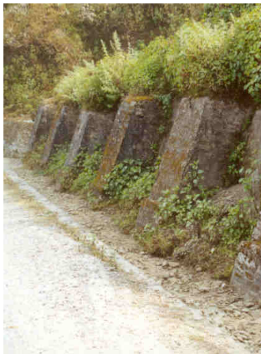
Buttressed mortared masonry wall
