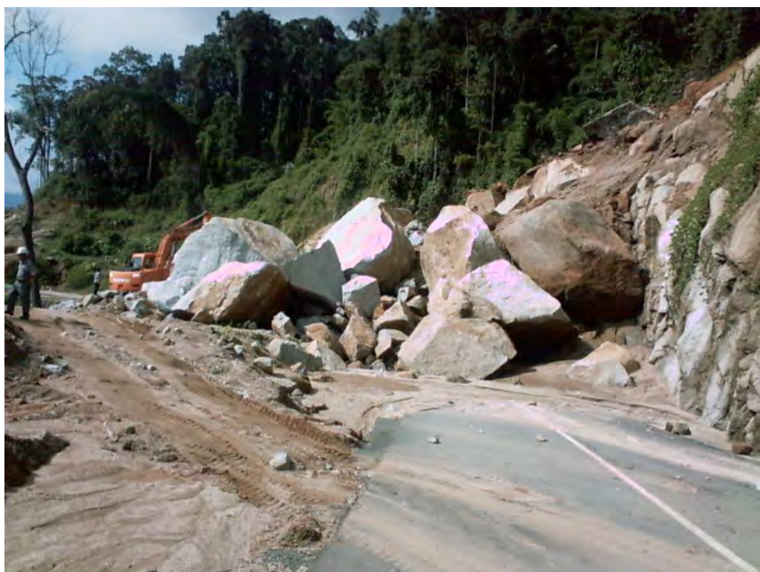
Figure 2-8: Rockfall on Road 18b
