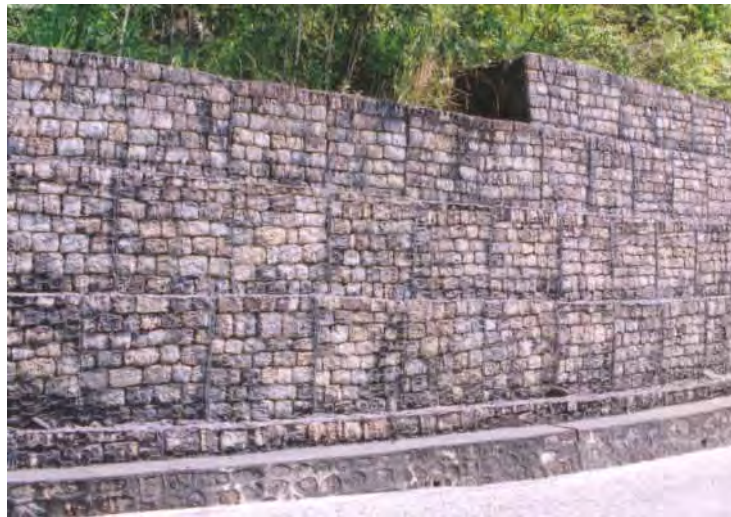
Figure 5-10: Typical gabion wall
