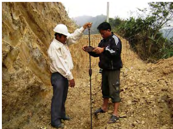
Figure 3-6: Dynamic Cone Penetrometer test
