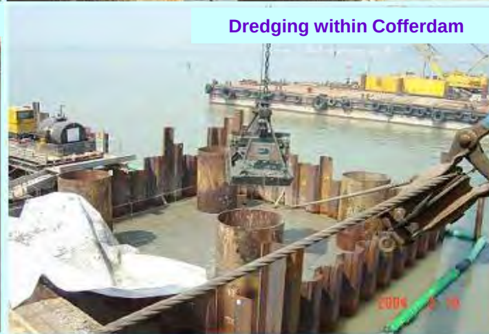
Cofferdam for pile cap construction
