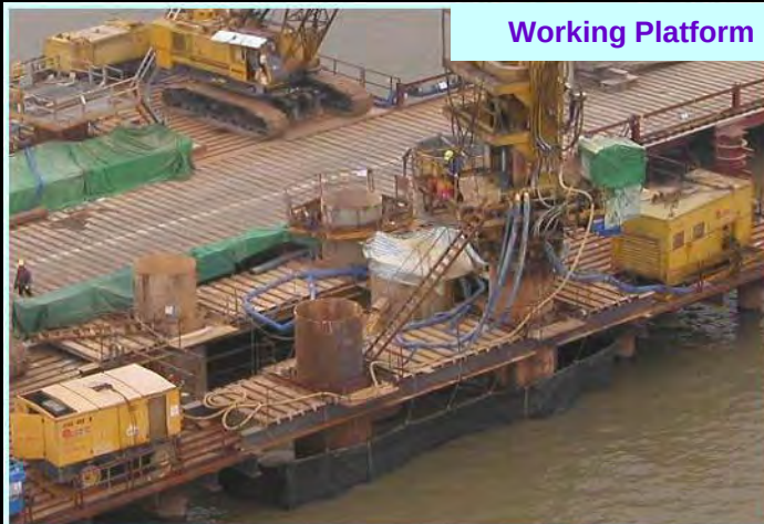
Cofferdam for pile cap construction
