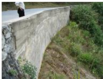
Reinforced concrete wall
