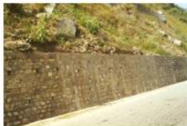
Mortared masonry wall
