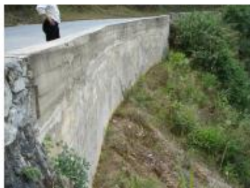
Reinforced concrete wall
