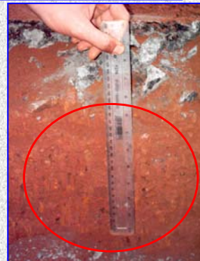
Poor gravel in placed in 1 layer? (specified 2)
