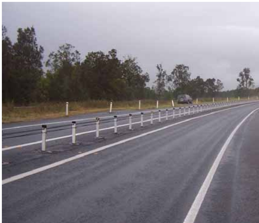
Figure 2: Centre-of-road wire rope barrier, NSW
