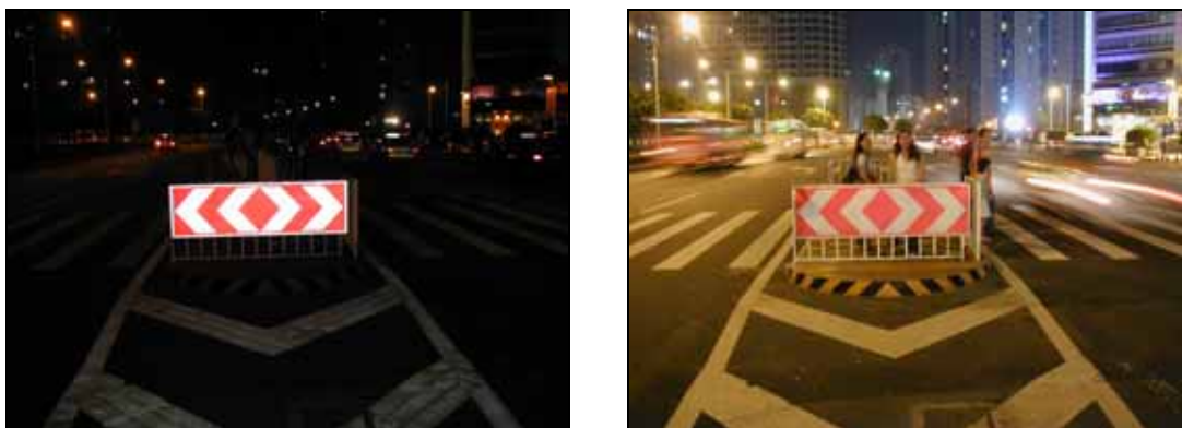
Figure 9 Pedestrian refuge island, with and without lighting, Guangzhou. Photos by Michael King.
