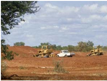
Re-instatement operations in a borrow pit.
