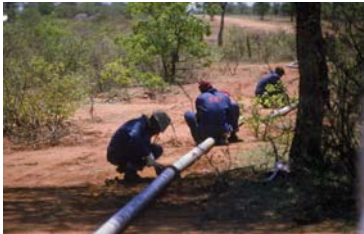
Supply of construction water may involve establishing large temporary pipelines.
