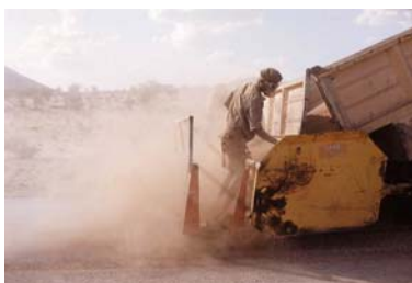
High contents of dust and fines in the aggregate is more critical for performance of a surface dressing than an Otta seal.
