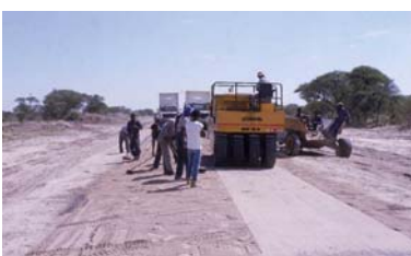
Rolling of sand seal.
