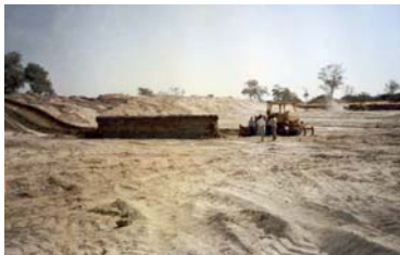
Large thickness of overburden does sometimes exclude labour-based methods for winning gravel materials (the example shown in the picture is from construction of LVSRs where the thickness of the overburden is in excess of 2m).
