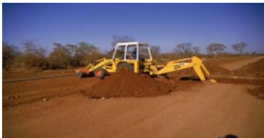
Excavators are convenient for various applications, including lifting.
