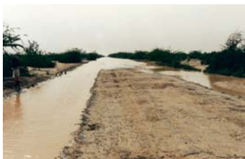
Overtopping on LVSRs, although undesirable, has less impact on the economy than if it occurs on HVRs.
