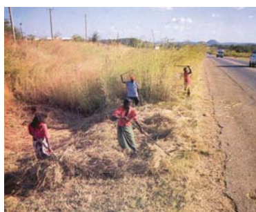
Grass cutting – a typical, labour-based, routine maintenance activity.
