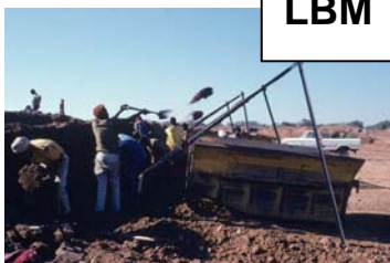
Screening aggregate by labour-based methods into tractor buckets (Otta seal is shown, sand seals would be similar).
