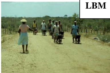
Wheelbarrows constitute part of the equipment used in LBM.
