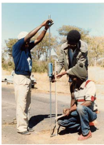
The DCP test in progress.
