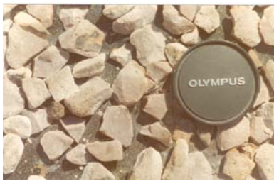
The need for cubical chipings is essential for good particle interlock in Chip seals.
