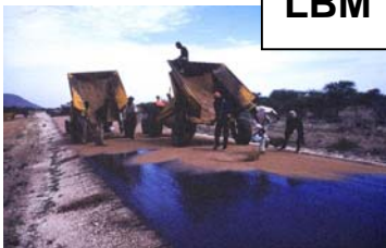
Spreading aggregate by labour-based methods from tractor buckets (Otta seal).
