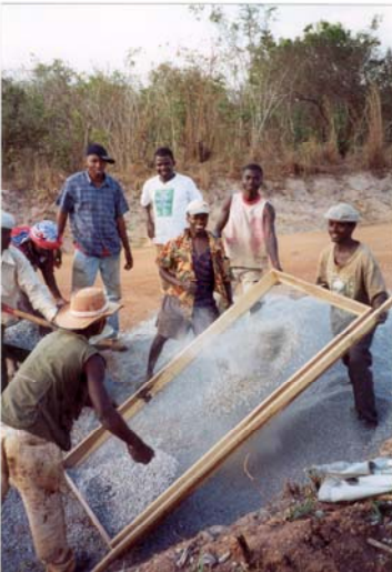
Screening of aggregate for road surfacing.
