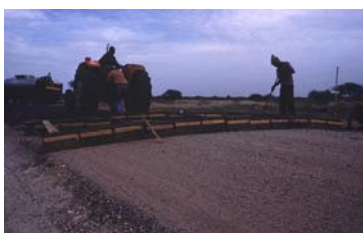
Drag brooming is sometimes applied in order to improve distribution of aggregate.
