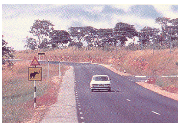
Typical LVSR offering many advantages over an unsealed road. In certain circumstances a bituminous surfacing may be warranted at traffic levels of less than 100 vpd.
