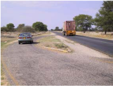
Lay-bys provide a safe haven where vehicles can pull off the road.
