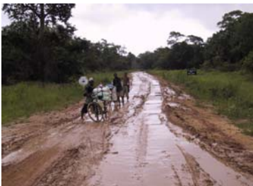
Trafficability of unpaved roads is adversely affected during the wet season.
