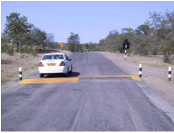
Well-designed speed humps are an effective means of slowing down traffic.
