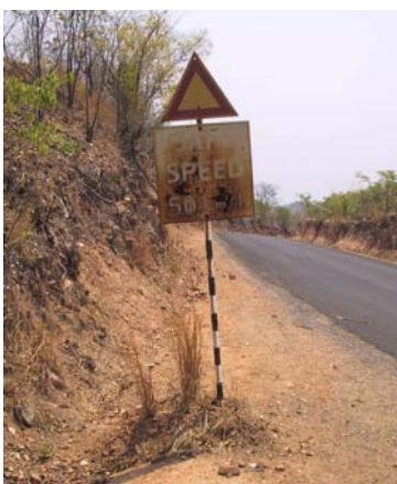
A poorly-maintained road sign can be the cause of road accidents.
