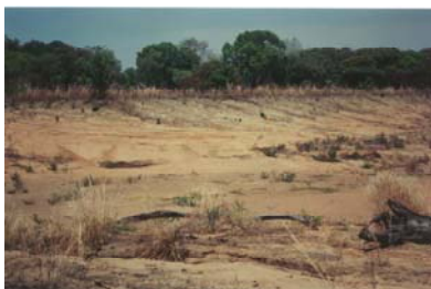
Un-renovated borrow area – typical of many countries in the SADC region
