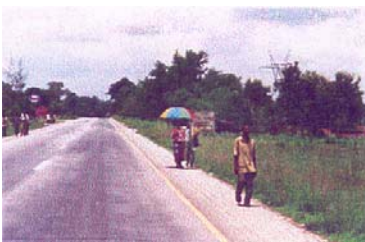
Where a segregated footpath is not possible, the use of relatively wide, sealed shoulders provides an acceptable surface for walking or cycling.
