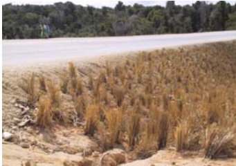
Bio-engineering offers the engineer a new set of tools, but does not normally replace the use of civil engineering structures. The materials and skills are all available in rural areas, however remote.
