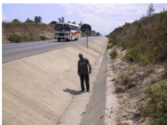
Deep V-type drainage ditches leave no room for recovery if a vehicle runs off the road.
