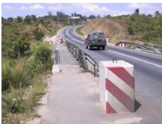
A segregated footway on a narrow bridge provides protection for pedestrians.
