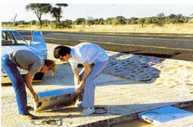
Installing portable weighbridge in pit
