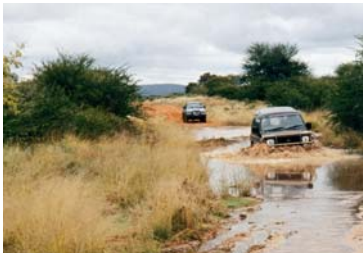
Short sections of road in poor condition can benefit significantly from spot improvement works.
