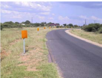
Additional signage should be provided on dangerous curve.
