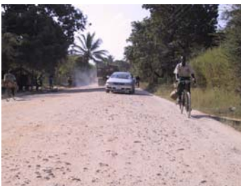
Due to loss of fines, gravel roads often become very rough which make driving conditions hazardous and, in addition to severe driver discomfort, impose very high vehicle operating
