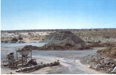
(a) Original pit used for construction.
