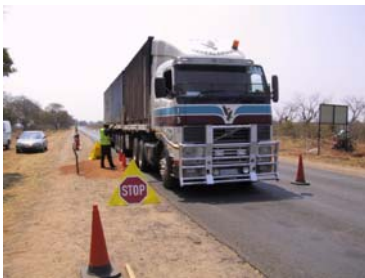
Axle load survey in progress. Such surveys are typically carried out over a 24 hour period for seven days.
