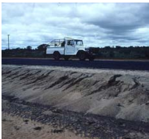
Severe erosion of side slopes that can lead to siltation of streams and rivers.
