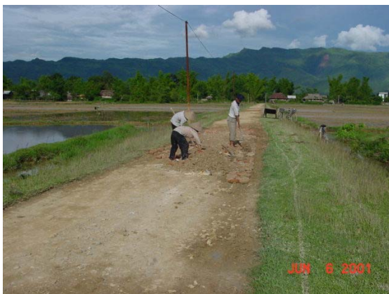
Figure 16 – Commune maintenance team involved in maintenance
