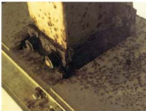
Figure 61 - Rusted/eroded steel
