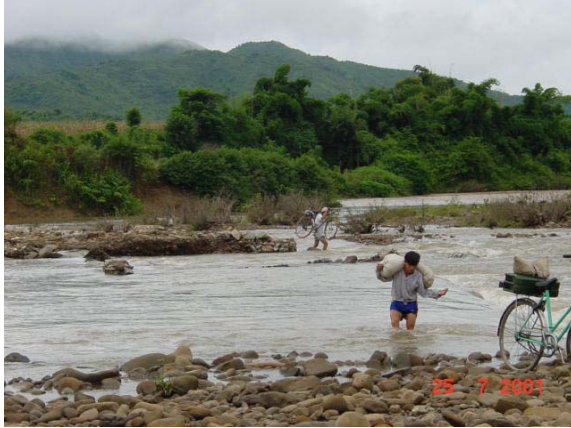
Figure 63 - Causeway washed out by flood
