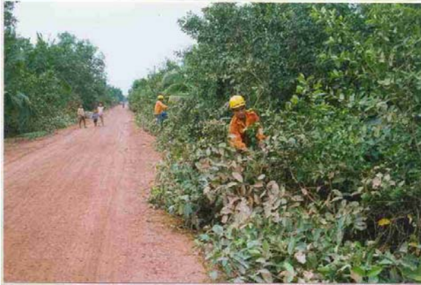
Figure 13 – Rural roads maintained by contractors
