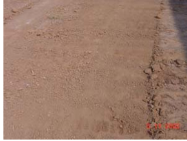
Figure 49 Surface before and after dragging by steel I beam
