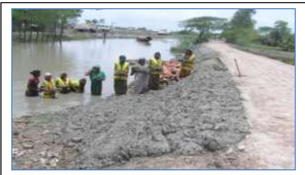
iii. LCS Member Repairing Shoulders
