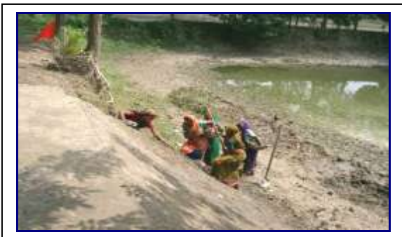
v. Repairing Road Side Slope
