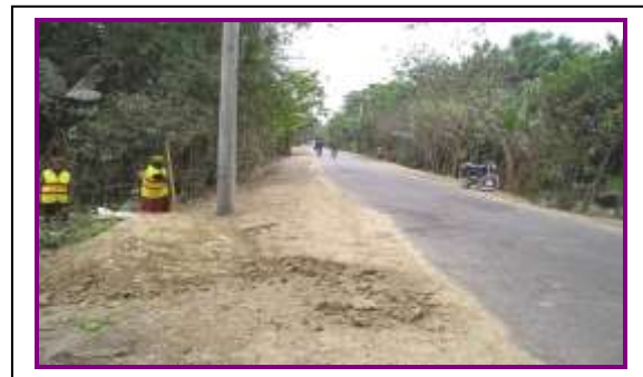
vi. Stockpiling Soil for Monsoon
