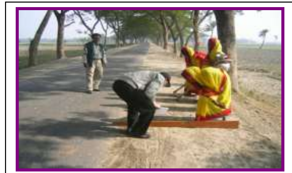
vi. LCS Member Repairing Shoulders
