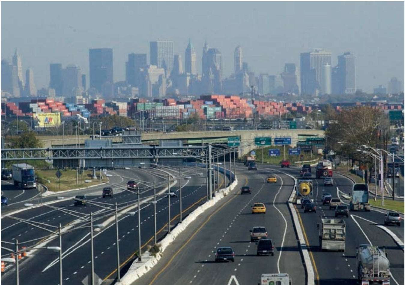
Truck lanes on the New Jersey Turnpike just outside of New York City.
