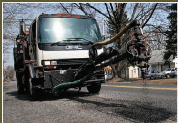
Courtesy of Patch Management Pothole Killers.
