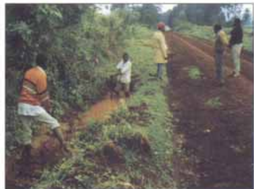
Labour Clearing Existing Drainage System
