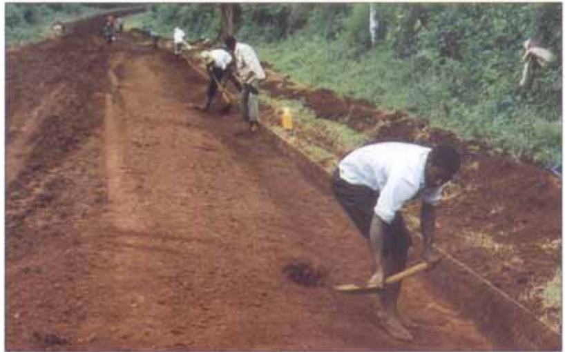
Labour Drainage Work
