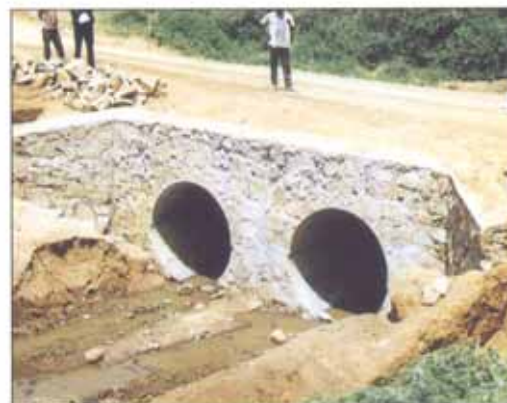
Culvert Rebuilding Work
