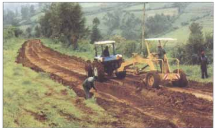
able to Rebuild the Road Camber
