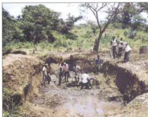
Culvert Excavation for a Spot Improvement
