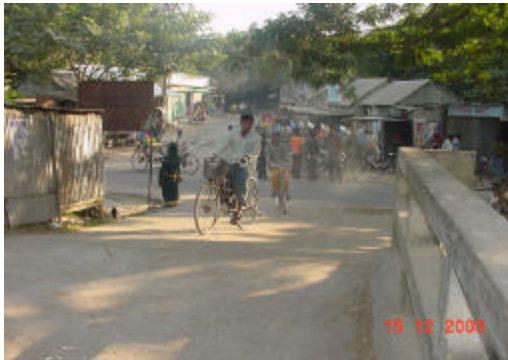
Intersection: accident black spot (a bridge with high gradient accessing the main road)
