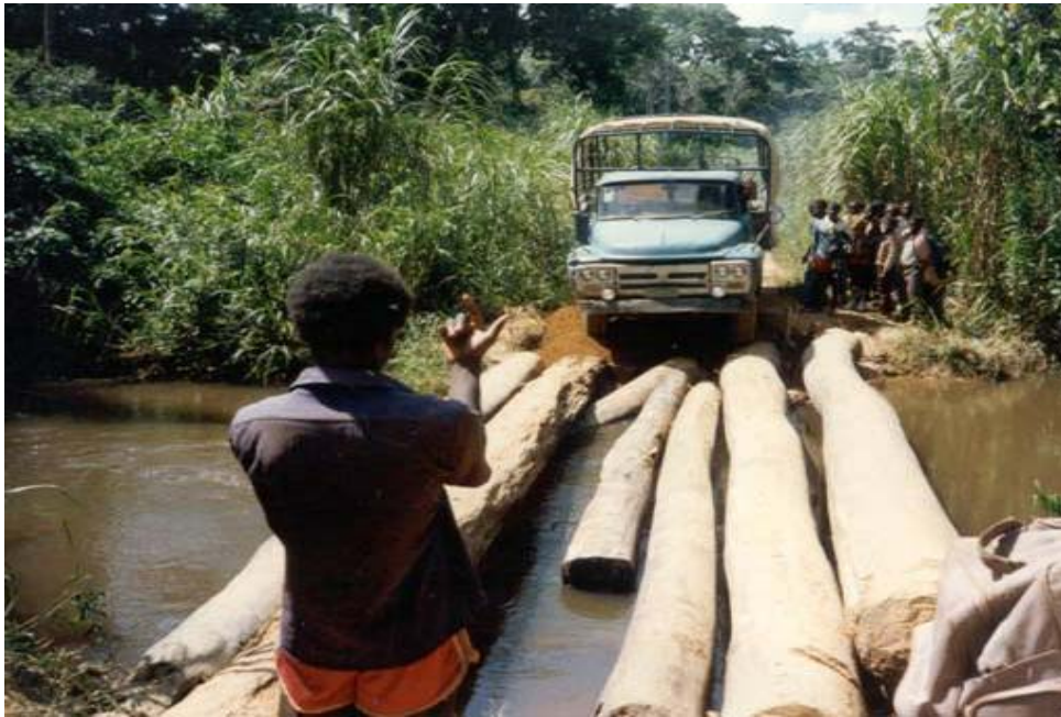
Lack of bridge provision by Rural Roads Offices in Kindu / East Congo (Local Self-help)
