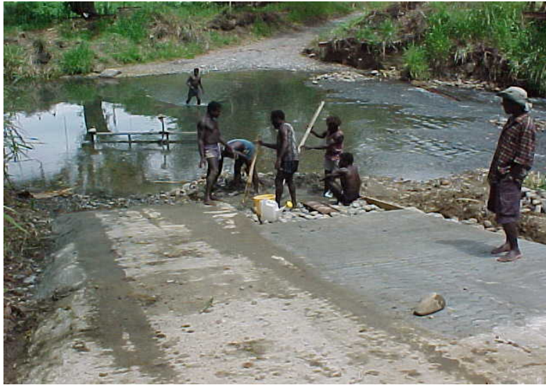
A community group constructing a Ford approach by CA, 2006
