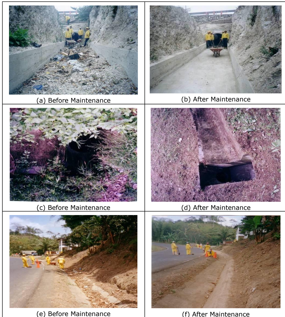
Figure 7. Example of drainage conditions before and after maintenance in the province of Manabi, Ecuador.
