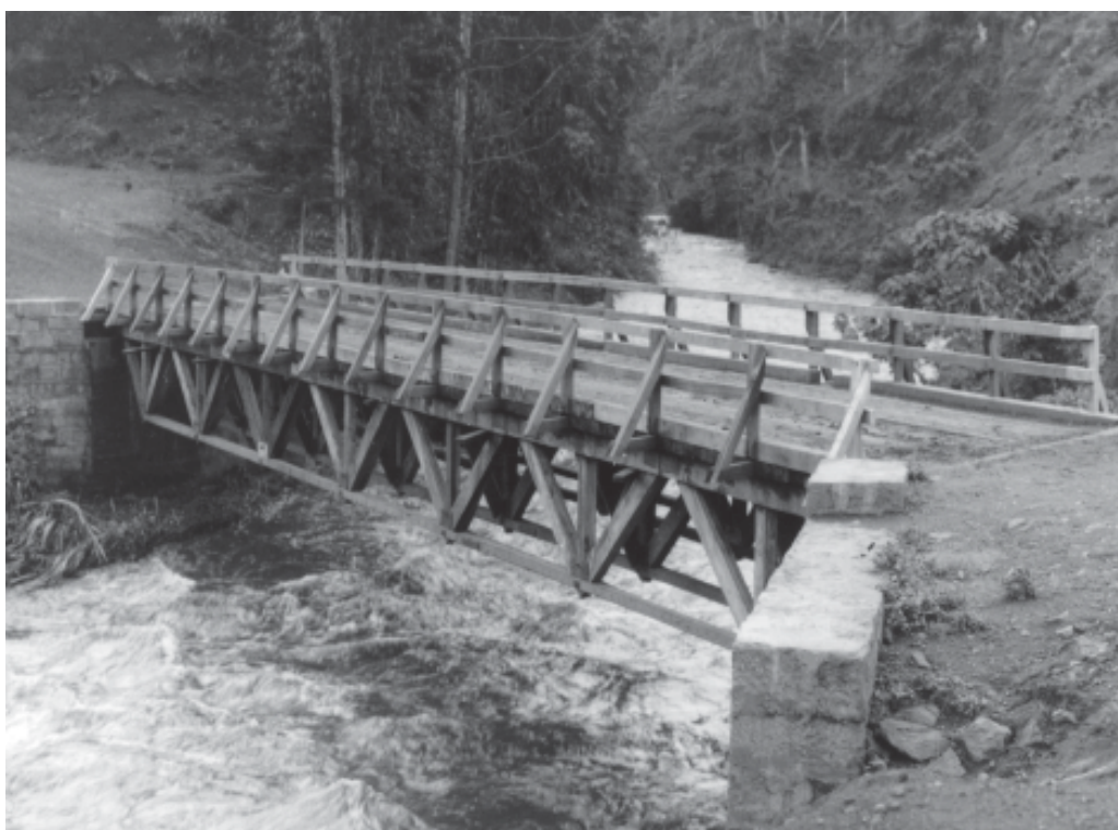
Figure 13.1 Timber panel bridge
