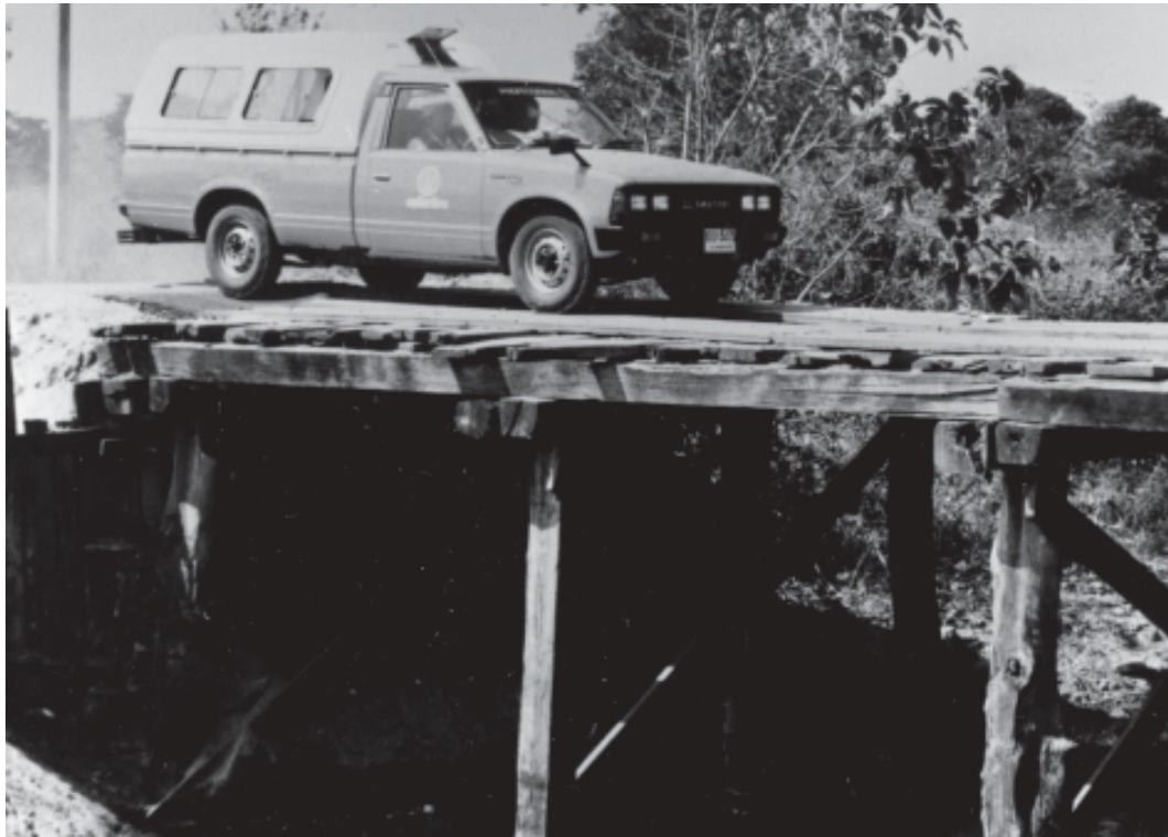
Figure 13.6 Timber deck on piled piers and abutments
