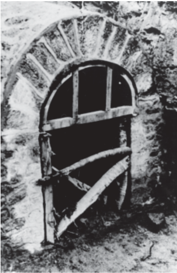
Figure 15.5 Masonry arch culvert with simple wooden formwork
