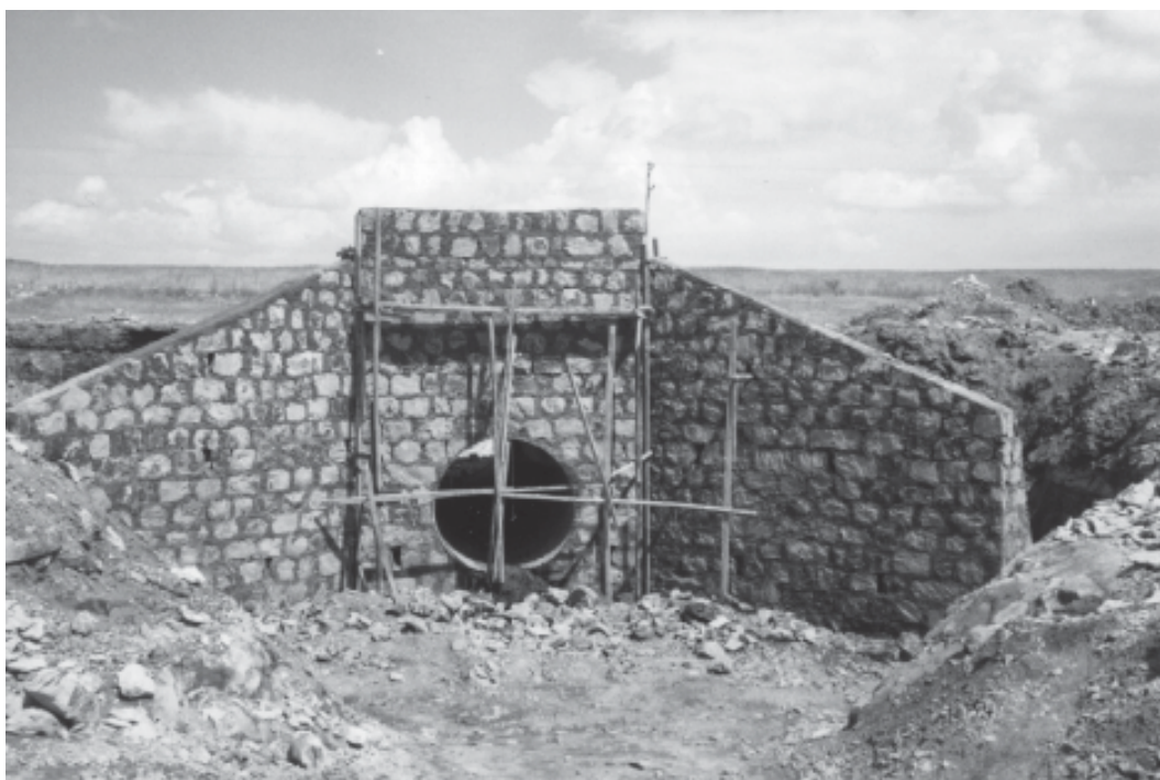
Figure 15.1 Culvert with masonry headwall and wingwalls
