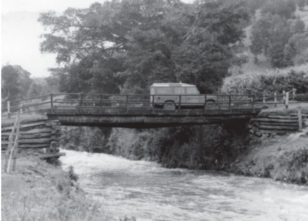
Figure 13.4 Log abutments with integral wing walls
