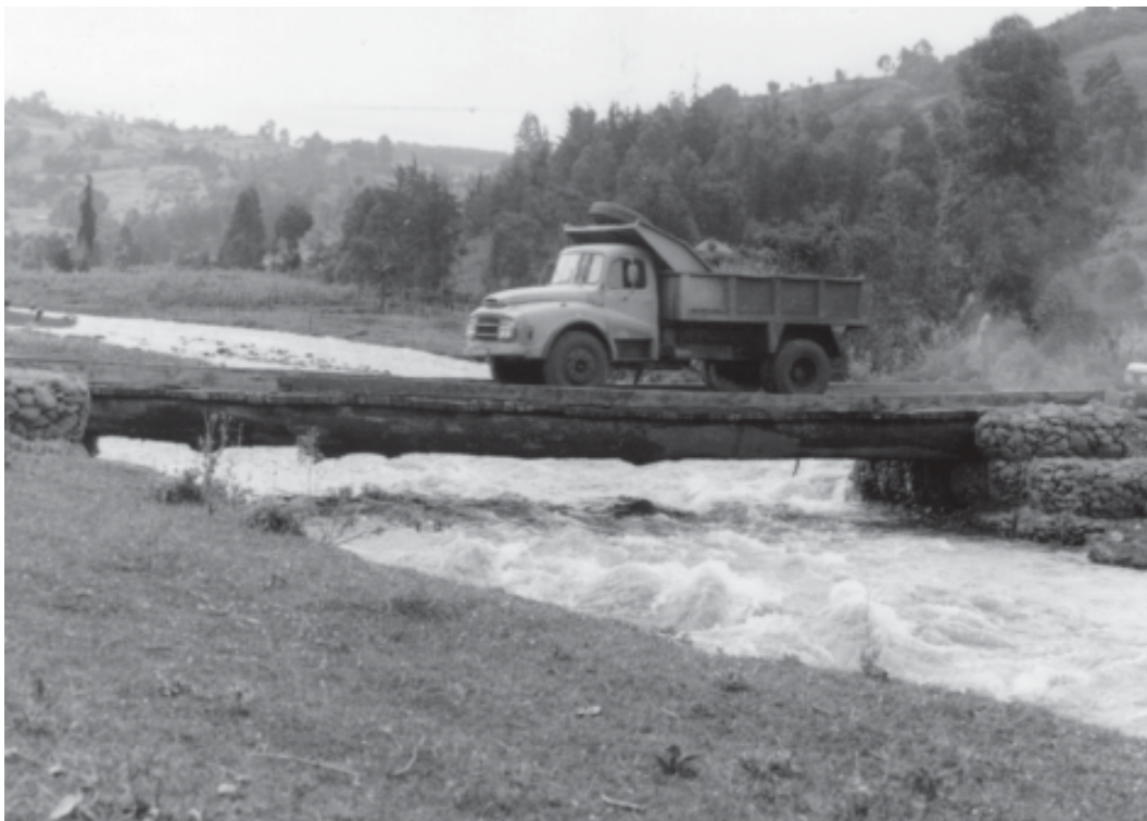
Figure 13.3 Temporary bridge on gabion abutments
