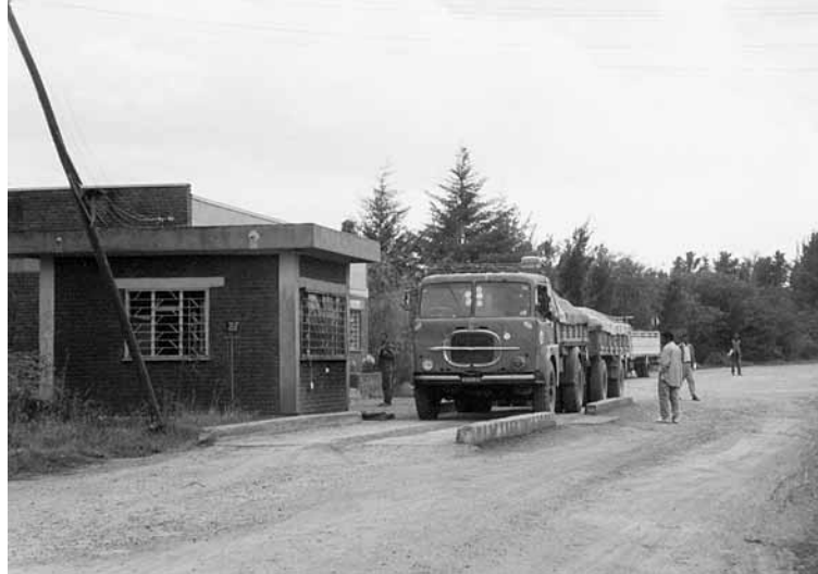
Figure 5a Fixed weighbridge site
