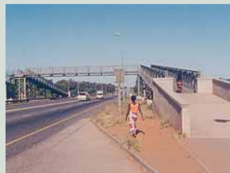
Figure 2.11 A pedestrian bridge enhances safety over this busy national road in Mozambique
