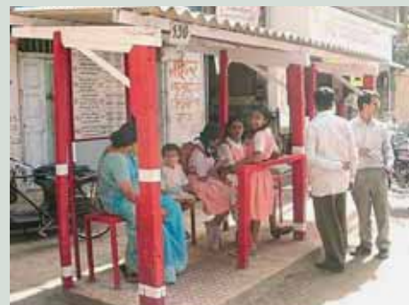
Figure 3.27 Upgraded bus stop showing colour contrast and seating in Pune
