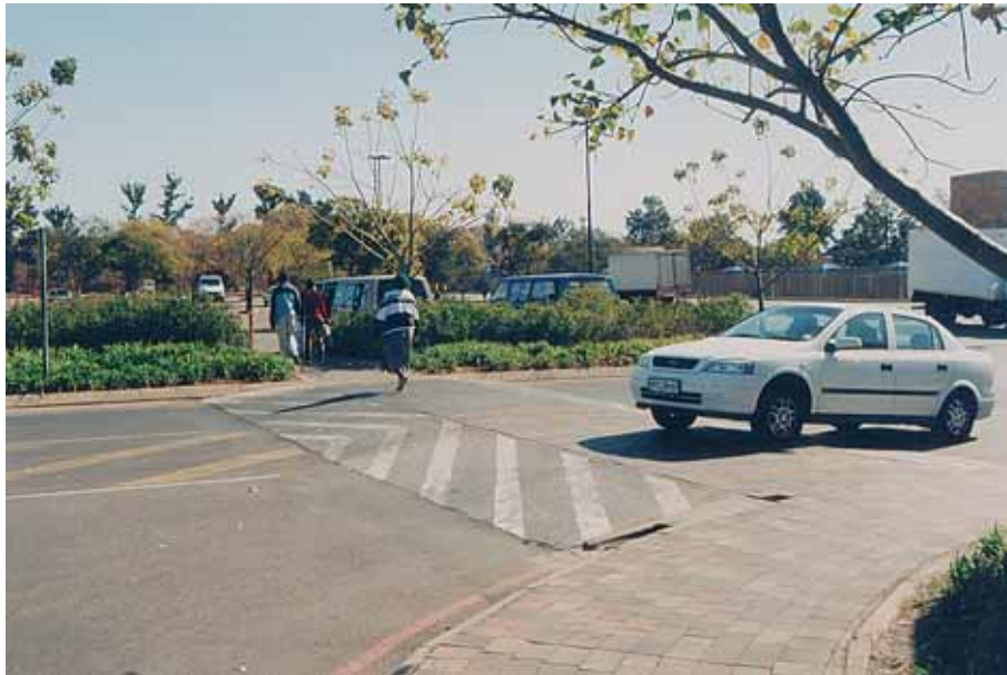
Figure 3.22 Raised crossings used judiciously can enhance pedestrian safety and accessibility
