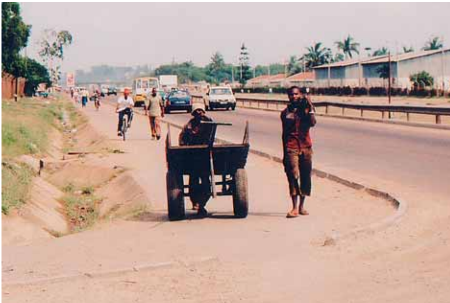
Figure 3.18 A pavement level with the carriageway but separated from it with a low kerb is easily constructed and provides access to all users
