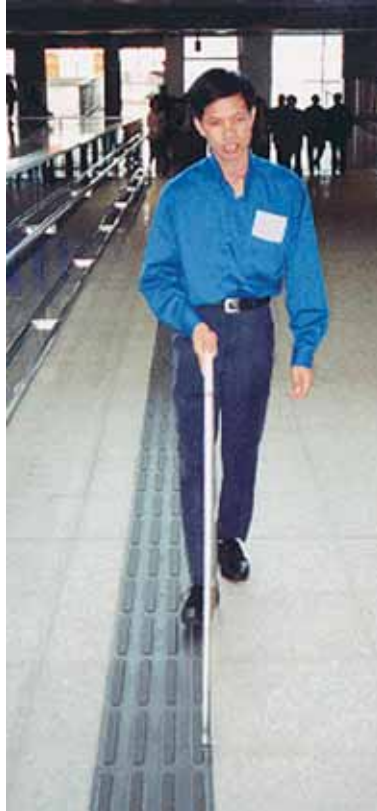
Figure 3.10 Long cane user following a guidance path (Source: Access Exchange International)
