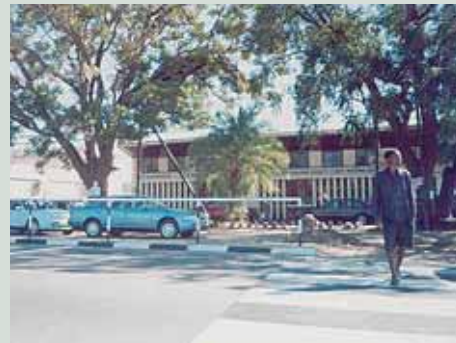
Figure 3.6 To enable passengers to safely cross the busy road to the hospital and the opposing minibus stop, a pedestrian crossing is installed with kerb ramps. Minibuses habitually block this section of road by drawing up over the kerb to load and unload passengers. The unsafe situation is rectified and ordered better through installation of a guardrail to prevent passengers from boarding anywhere outside the designated bus stop area.
