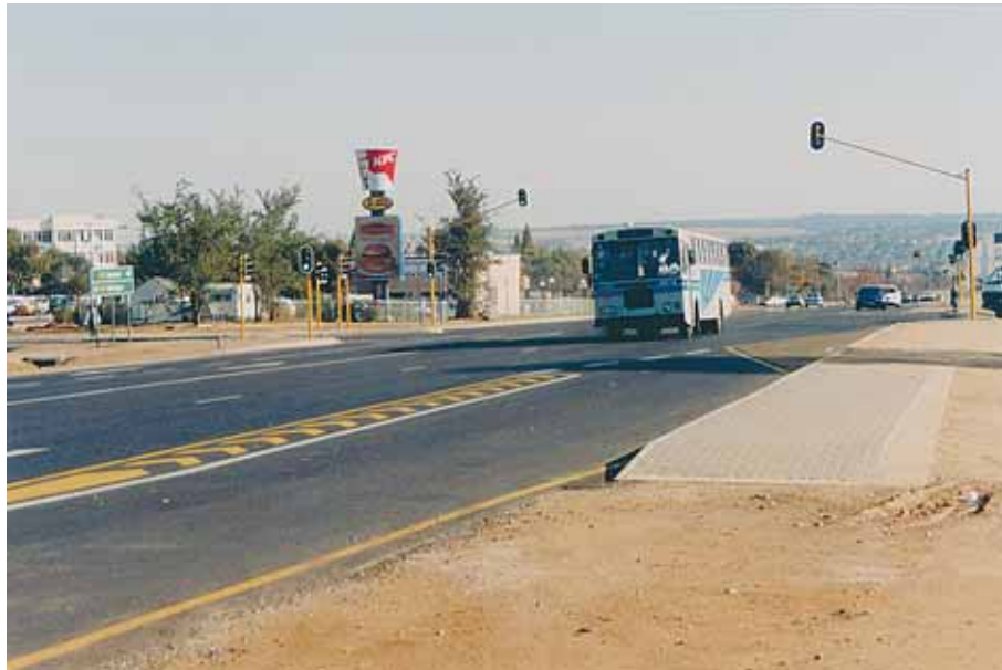
Figure 3.35 Safety and accessibility can be enhanced as a first step simply by providing a paved off-road boarding area for bus and taxi passengers
