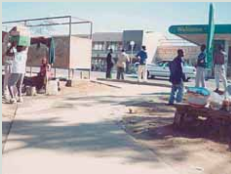
Figure 3.5 A new paved pedestrian footway is provided to ensure access for pedestrians and wheelchair users to the minibus stop. A new bus shelter, that is fully accessible to all users is under construction at the same site.
