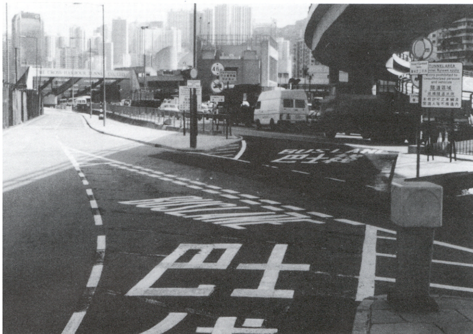
Plate 1 A bus gate providing buses with unhindered access to main road: Hong Kong
