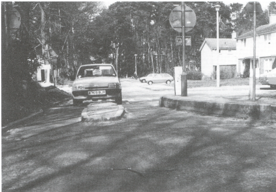
Plate 15 Busway entry barrier
