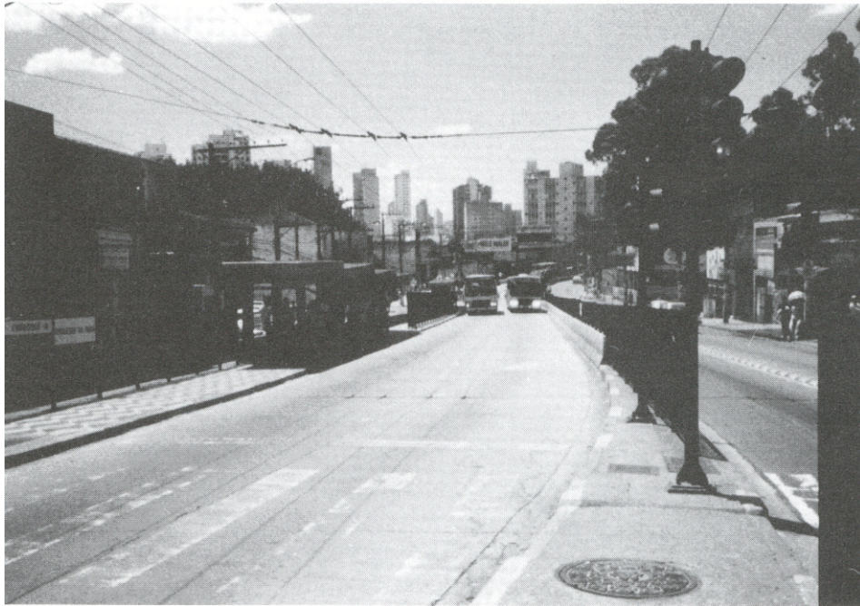
Plate 4 Busway transit stop, with overtaking facility: Sao Paulo
