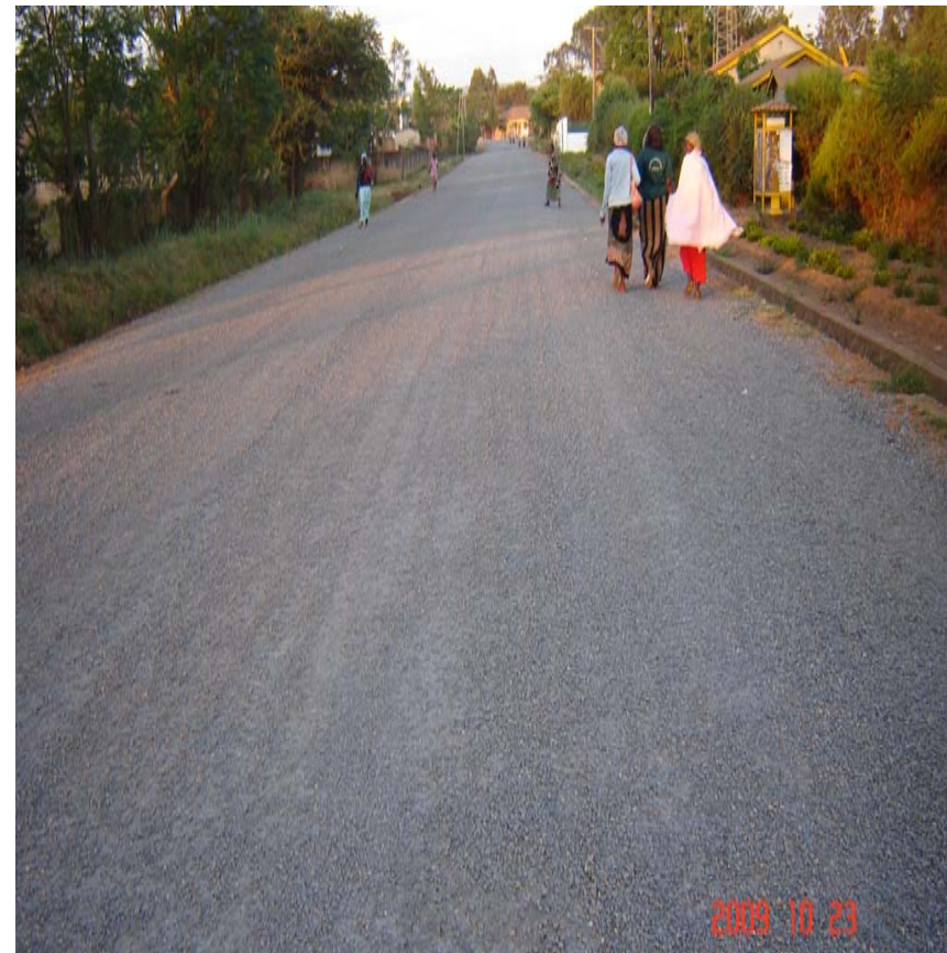
Photo 18 and 19: Conventional Bituminous Surface Dressing on Low Volume Regional and Urban Roads in Kagera Region (Left) and Rukwa Region (Right) Few Months After Construction
