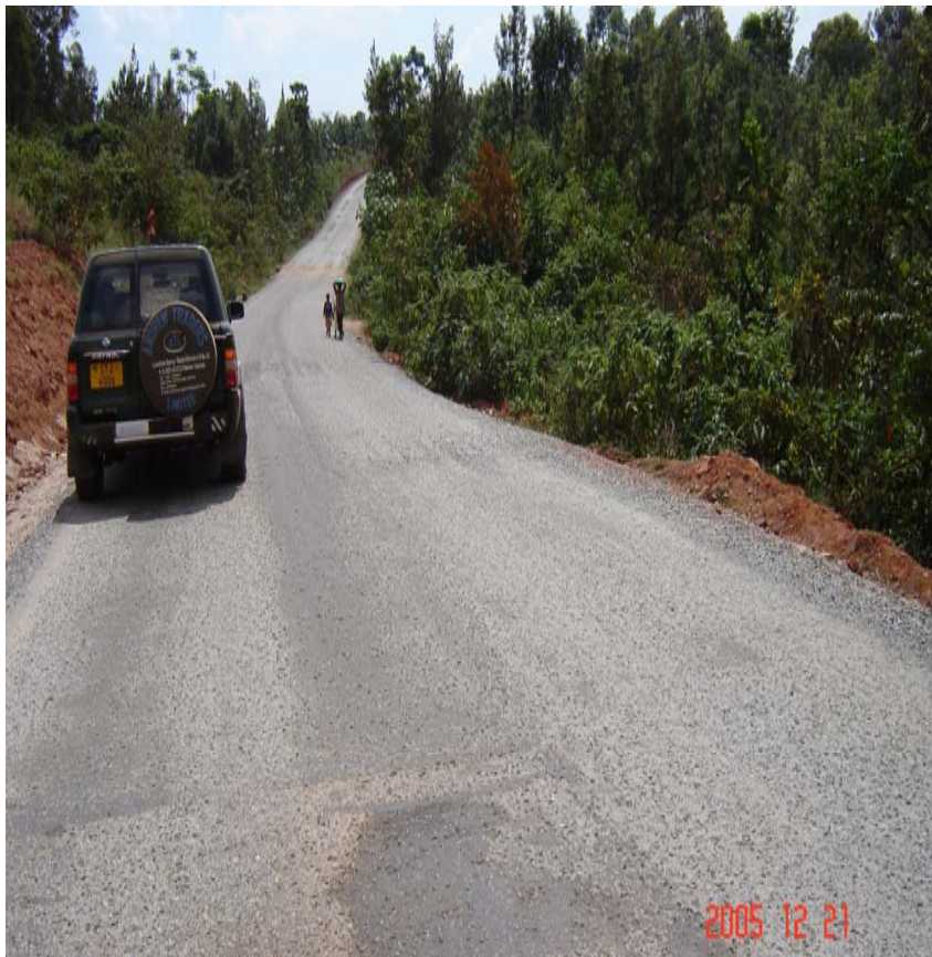
Photo 18 and 19: Conventional Bituminous Surface Dressing on Low Volume Regional and Urban Roads in Kagera Region (Left) and Rukwa Region (Right) Few Months After Construction
