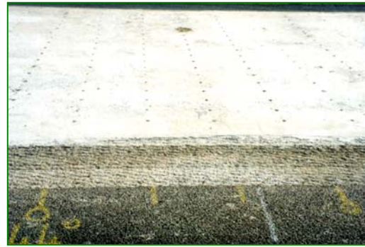
Figure 3 concrete slab of euphonic pavement
