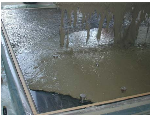
Figure 6 : UHPFRC casting.
