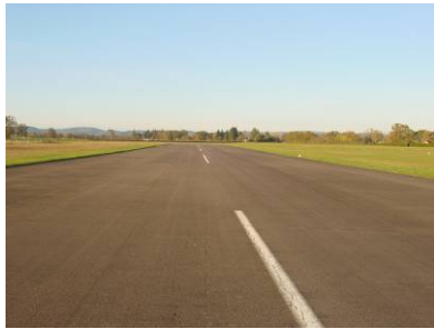
View of the airport test track Camera located on the axis
