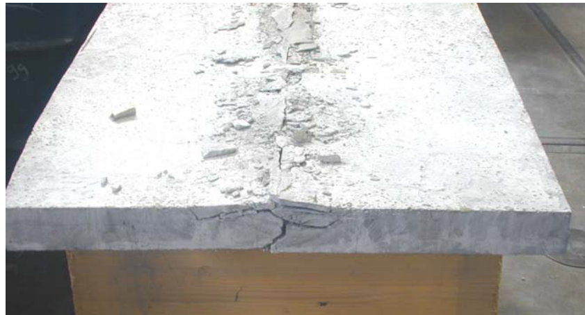
Figure 16 : Failure of the cold joint ( post mortem sawn cross-section)
