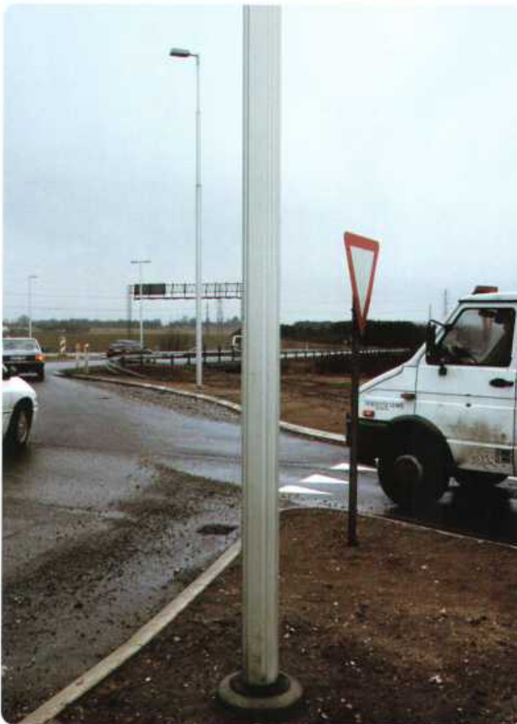
Frangible lighting column.
