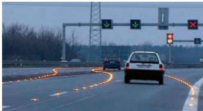
Figure 10.7. Tidal traffic flow system
