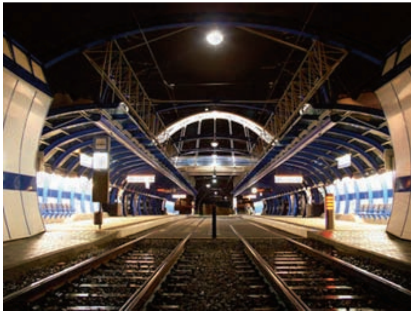
Figure 10.5. Separate tramway line in Prague
