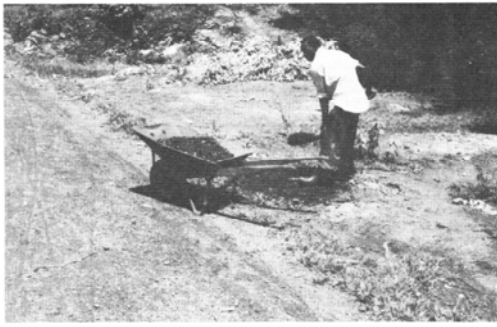
FIGURE 7 Excavating gravel for patching.
