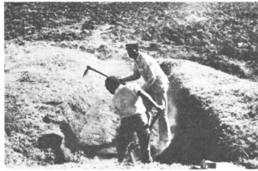
FIGURE 10 Cleaning culvert inlet.
