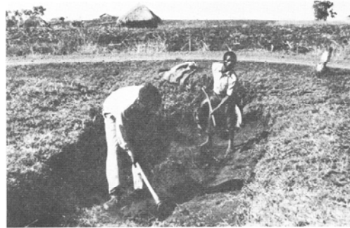
FIGURE 9 Cleaning culvert outlet.
