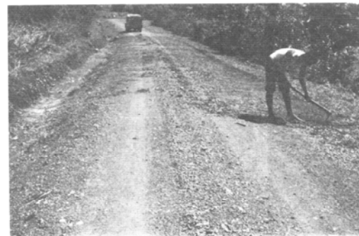
FIGURE 6 Grubbing edge.
