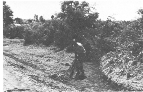
FIGURE 11 Cleaning miter drain.
