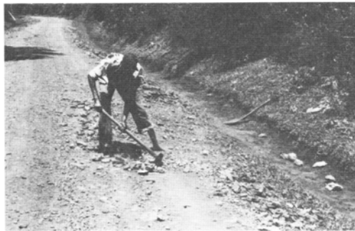
FIGURE 8 Reshaping carriageway.
