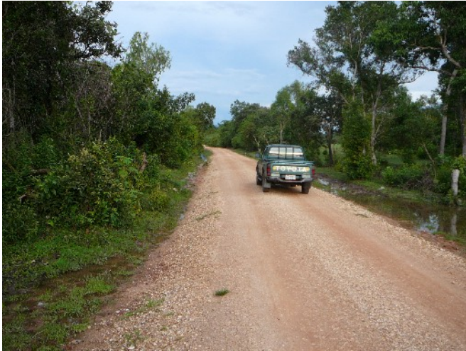
Typical low volume rural road in Lao PDR
