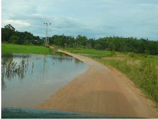
Flooding covering a rural road
