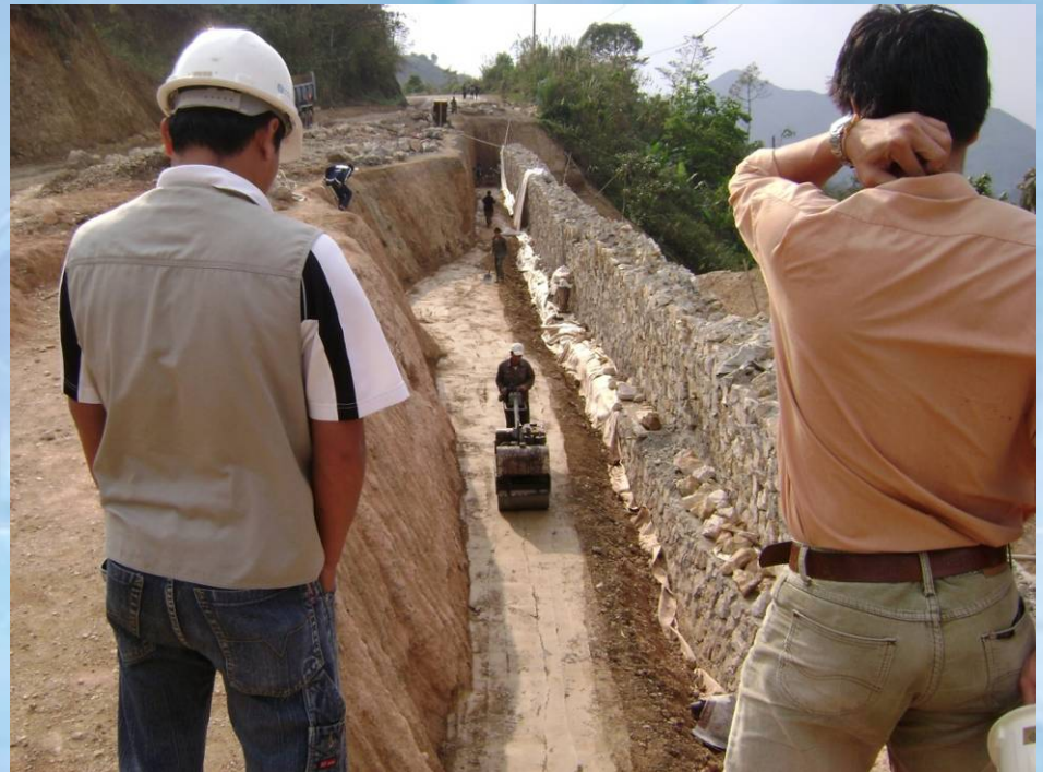
Compaction using pedestrian roller
