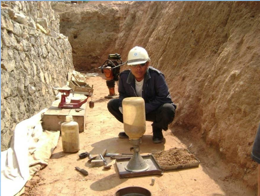
Backfill density testing
