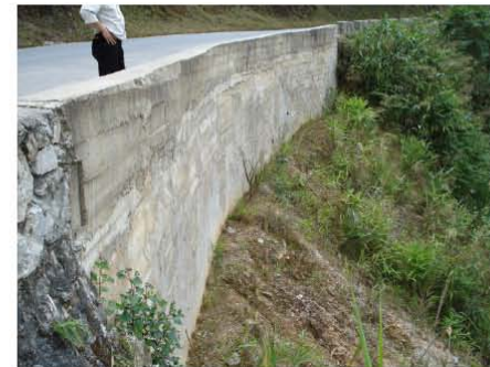
Reinforced concrete wall
