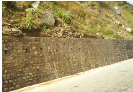
Mortared masonry wall
