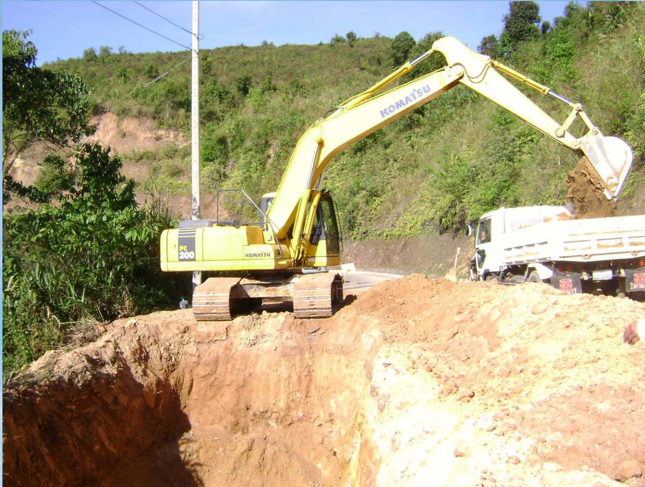
Removal of spoil
