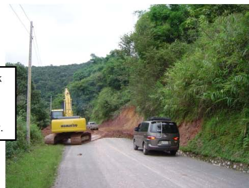
Emergency work following the collapse of a culvert on a national highway.
