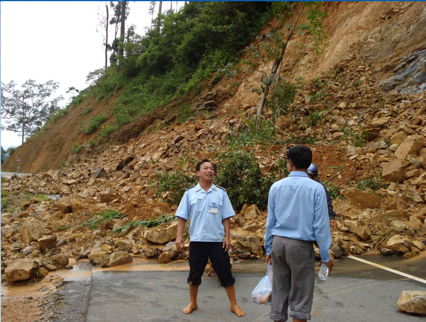
Typical above-road failure
