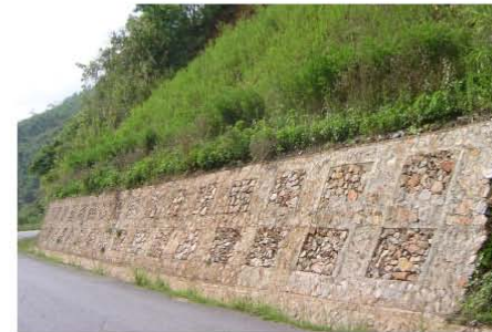
Composite masonry wall
