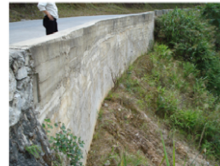
Reinforced concrete wall
