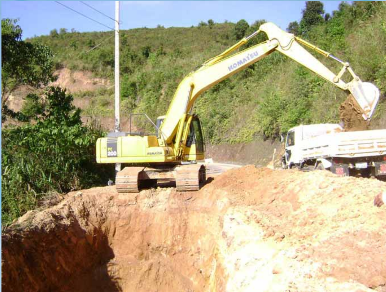
Removal of spoil
