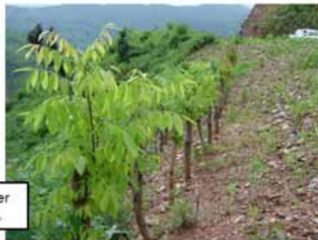
Road 13 North, km 316. A revetment wall and various types of bio-engineering works were used to protect the slope.
