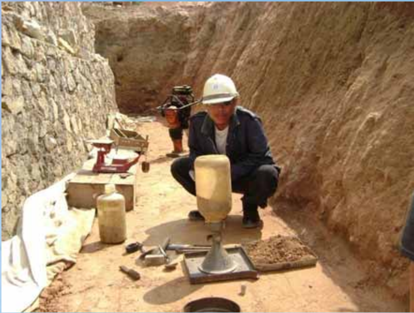
Backfill density testing
