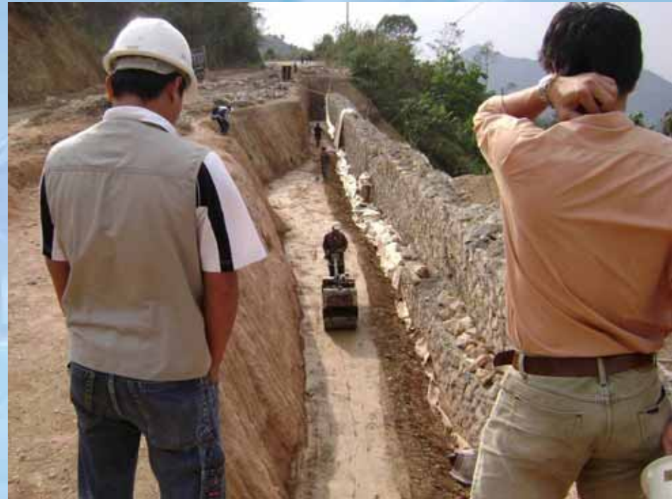
Compaction using pedestrian roller
