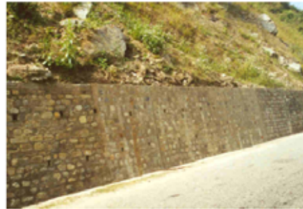
Mortared masonry wall
