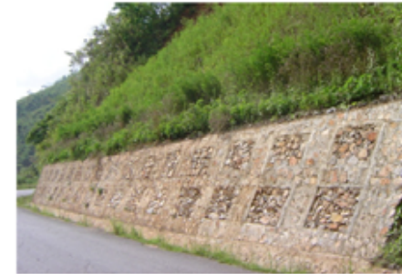
Composite masonry wall
