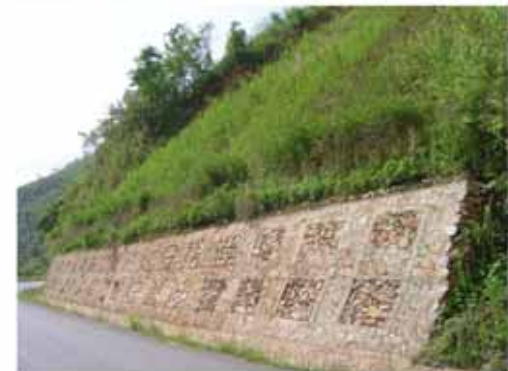
Road 13 North, km 316. A revetment wall and various types of bio-engineering works were used to protect the slope.
