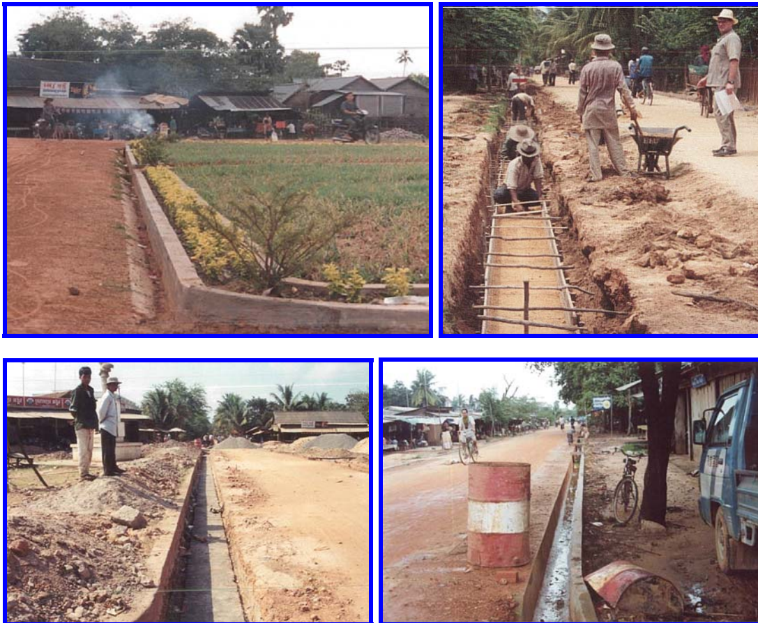
Images 20 - 23: Drainage Works
