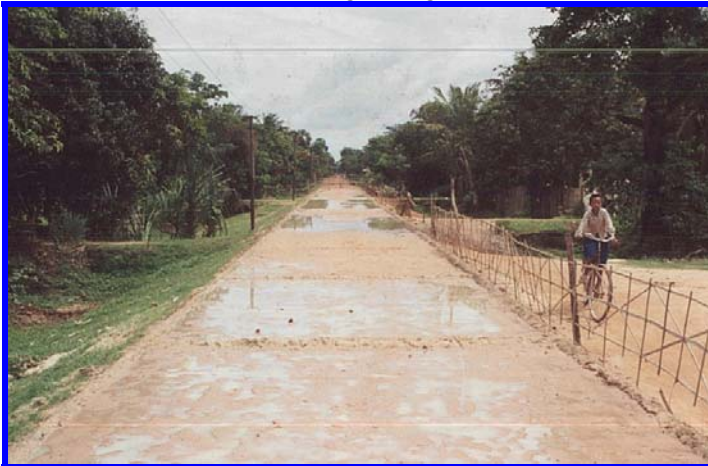
Image 19: Curing and Protection of Concrete
