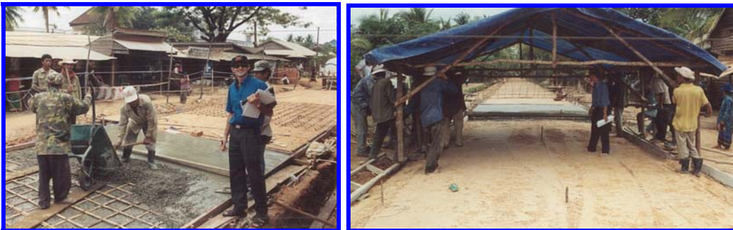
Images 14 & 15: Placement of Concrete and Sun Shelter
