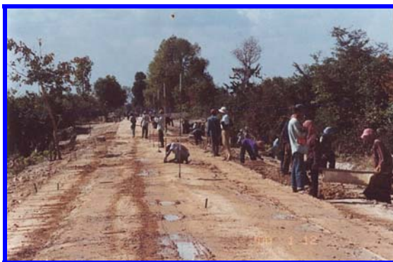
Image 9: Setting out of road alignment and level
