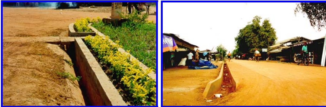
Images 5 & 6: Side Drainage Arrangements
