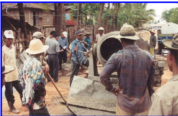
Image 13: Mixing of Concrete
