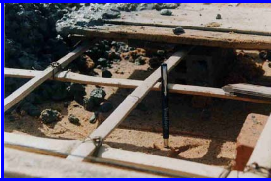
Image 7: Bamboo mesh located 5cm below finished slab level
