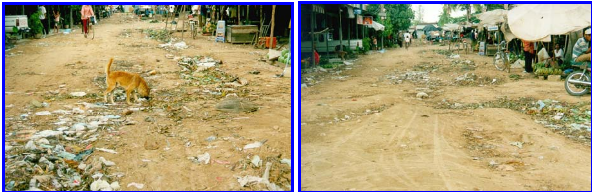
Images 3 & 4: Puok Market roads condition before construction
