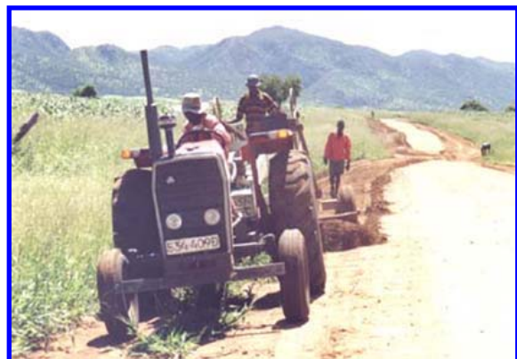
Figure 4 – Tractor towed grading
